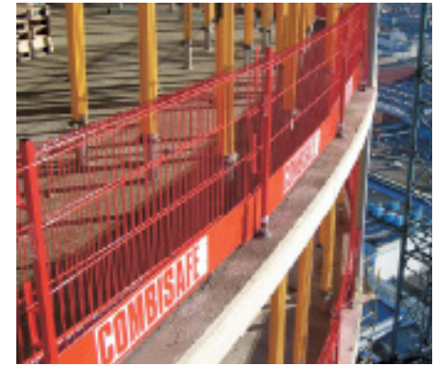
Sockets in slabs for edge panels
