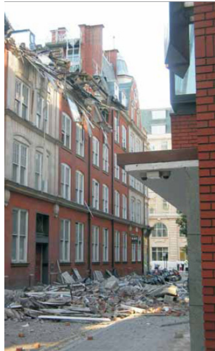
Dean Farrar Street building collapse (street view)
