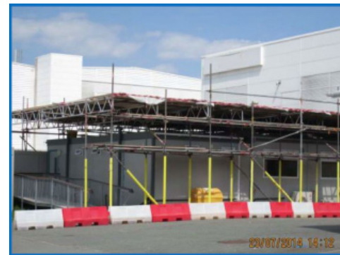
Design Scaffold Over the Office
