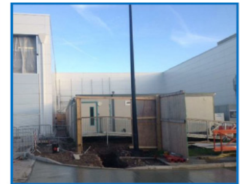
Completed Adjacent Structures
