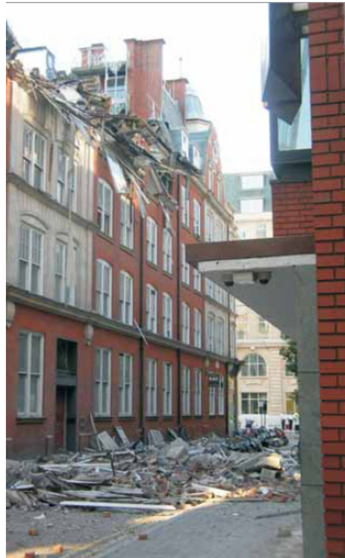
Dean Farrar Street building collapse (street view)
