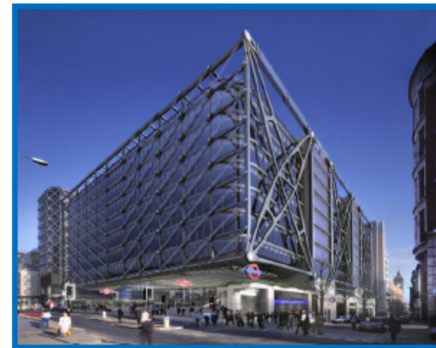
Cannon Place Bridge Structure
