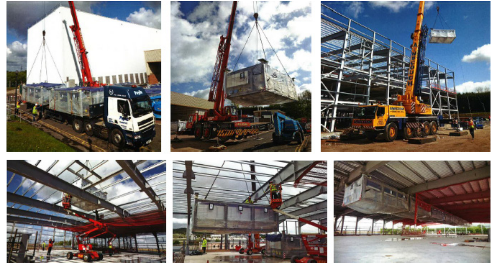
Module delivery and installation
