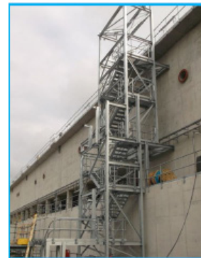
Erected Stair Units
