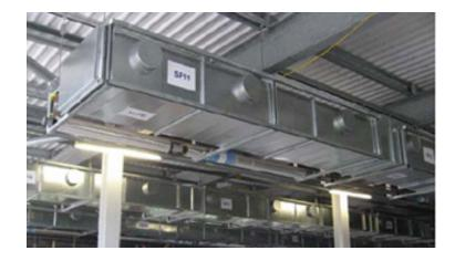
Fitting 200 pre-fabricated multiservice spines 6000mm long x 1500mm wide.
