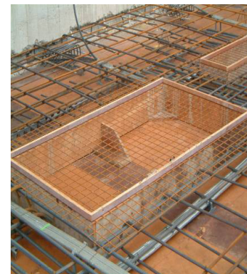
3. Small metal mesh prevents falls in open areas
