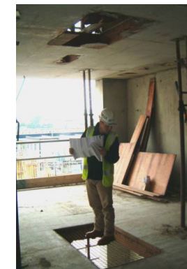
3. Small metal mesh prevents falls in open areas
