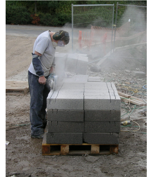
Avoid unnecessary or excessive cutting
