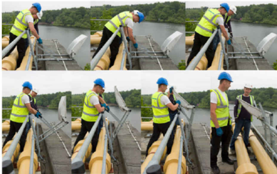
Bracket being unbolted and manoeuvred back into maintenance position
