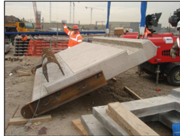
Temporary turning plates fitted to a precast panel.
