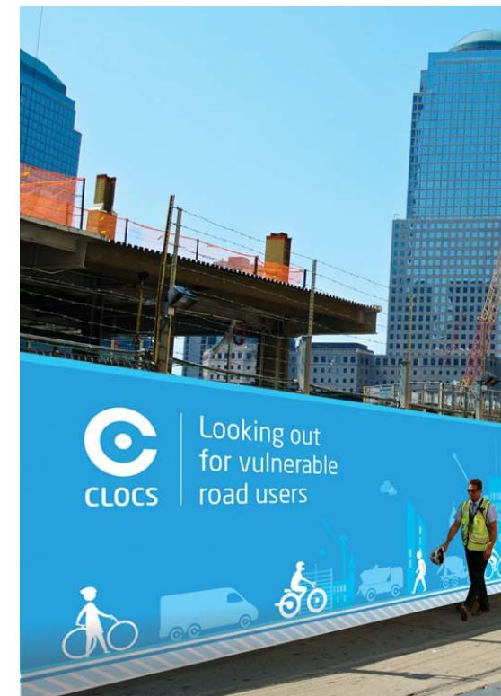
Example site hoardings
