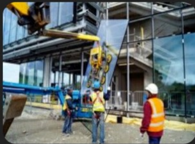
LIFTING HEAVY CLADDING
