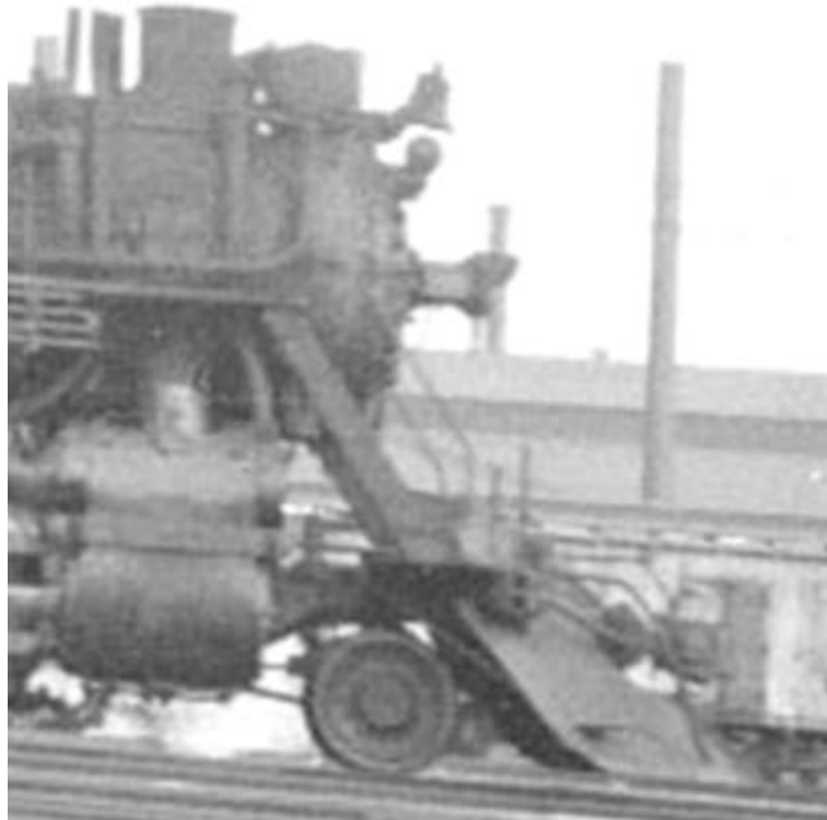
The thing's huge, and requires a completely new coupler and draft gear box! I've got other photos of 669 before it was wrecked in 1949, and the engine had a more conventional sheet steel pilot.
