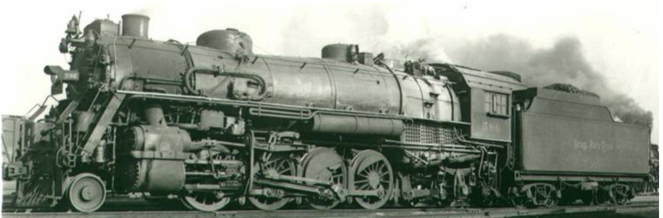
NKP 586, Madison, IL, 1938. This how the H-6o's looked with both the deck mounted air pumps and the feedwater heater added.
