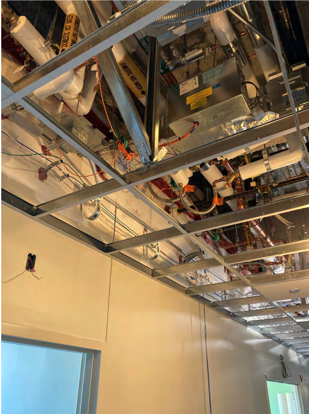
GRIDLOK® installed with Advancespan™ showing the compression post and one brace.
