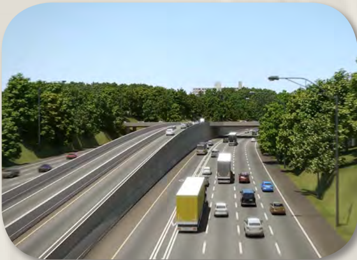
HOV-only interchanges and ramps are proposed at several locations on I-65 to improve access to the proposed HOV lanes.
