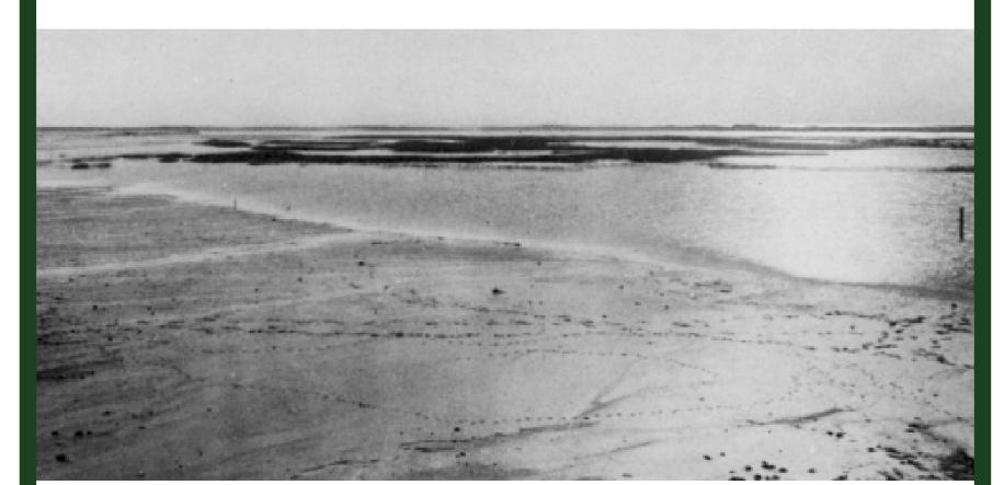
Herculean task of constructing the Lido course is gained from this photograph which shows in the cement of the filling process by pumping sand and the water of the lagoons which is now all hard gr
