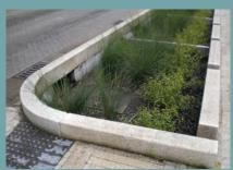
A rain garden works by capturing stormwater to irrigate plants, while at the same time reducing runoff and filtering the water.
