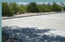
Pervious pavement is an effective way to reduce runoff where hard surfaces are needed. Perviou pavement does require periodic maintenance to preserve its porousness and effectiveness.
