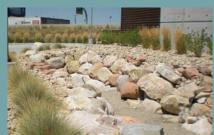
Landscaping can creatively incorporate detention basins to reduce runoff and filter stormwater.
