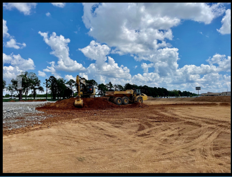
Pictured Left: Thompson Machinery Mass Grading Murfreesboro, TN
