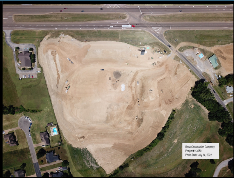
Pictured Left: Lauderdale County Hospital Site Work Ripley, TN
