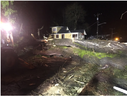
Where the fallen tree landed.
