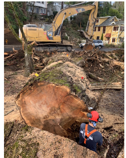
Removing sections of the fallen tree with an excavator.
