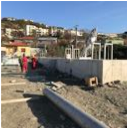
Photo 127. I-17 Gramsh wastewater treatment plant under construction (2)
