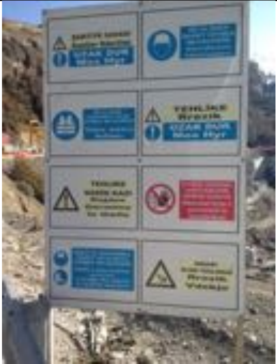
Photo 87. I-12 Safety signage at entrance to Moglicë work site
