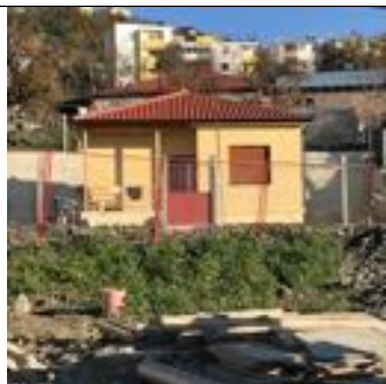
Photo 46. I-10 A replacement House in Gramsh
