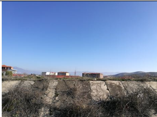
Photo 61. I-10 Residential Buildings to the West of the Resettlement Site
