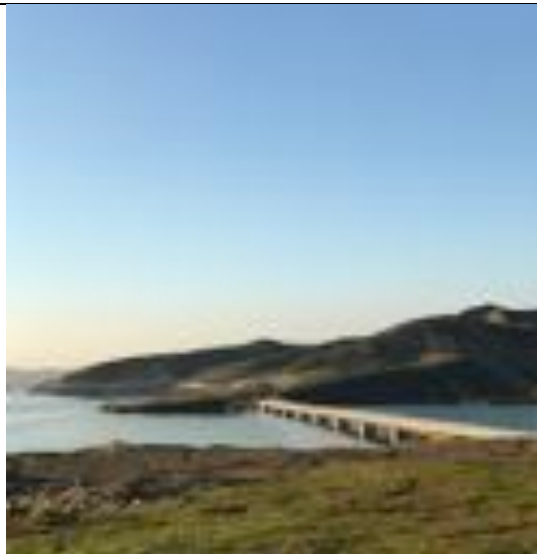
Photo 27. I-7 Example of a bridge crossing the reservoir, part of the north shore Banje-Gramsh replacement road
