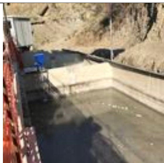
Photo 133. I-18 Sediment pond at Moglice tunneling site
