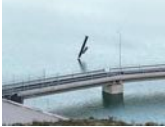
Photo 107. I-16 Pipe for flushing sediment with 'sedicon' technology, in centre of photo
