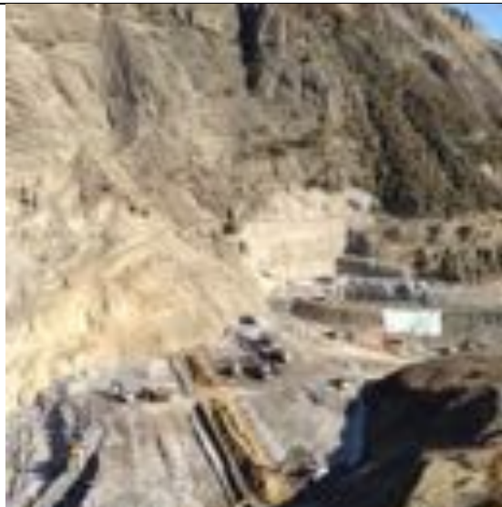
Photo 21. I-5 Work on Moglicë coffer dam.jpg
