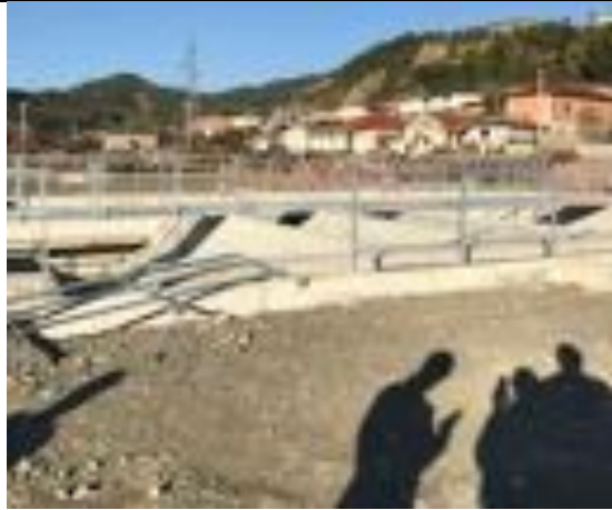
Photo 126. I-17 Gramsh wastewater treatment plant under construction
