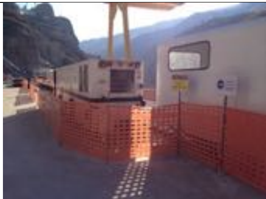
Photo 85. I-12 Restricted access to tunnel train
