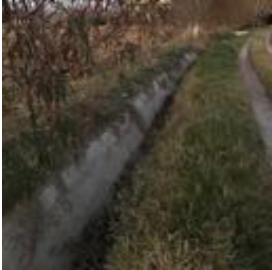
Photo 29. I-7 An irrigation channel, part of the rehabilitated irrigation scheme at Shushice
