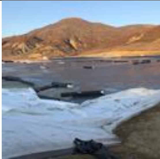
Photo 138. I-18 New landfill under construction at Maliq
