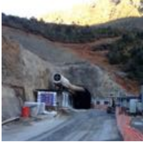
Photo 92. I-12 Tunnel access with ventilation
