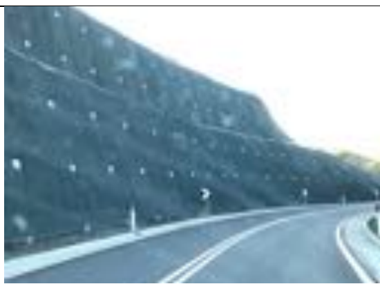
Photo 118. I-16 High-specification erosion protection used along replacement roads
