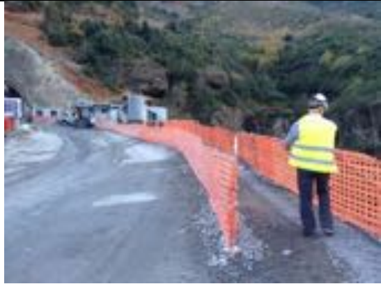
Photo 88. I-12 Separated tunnel access for vehicles and pedestrians
