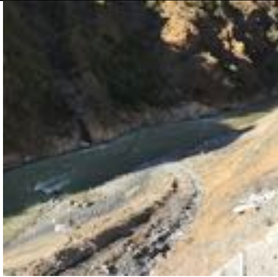
Photo 155. I-20 Devoll river at the approximate location of the Moglice powerhouse tailrace
