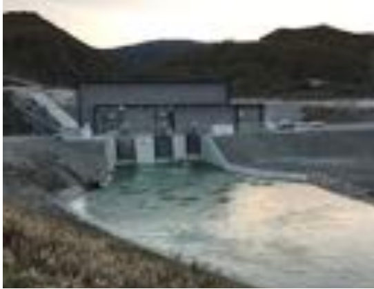
Photo 150. I-20 Tailrace of the Banje powerhouse
