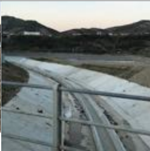
Photo 152. I-20 Emergency outlet channel at Banje
