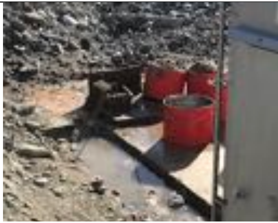
Photo 140. I-18 Sewage leaking or overflowing from Arsimak plants, with sludge gathered in drums
