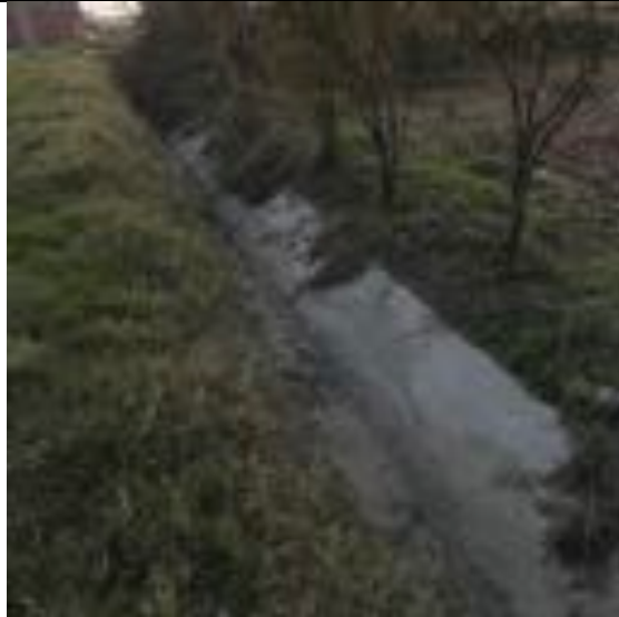
Photo 30. I-7 An irrigation channel, part of the rehabilitated irrigation scheme at Shushice
