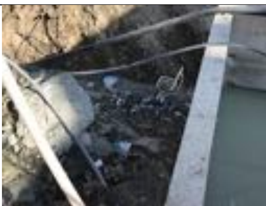
Photo 136. I-18 Trash disposed of beside creek behind sediment pond
