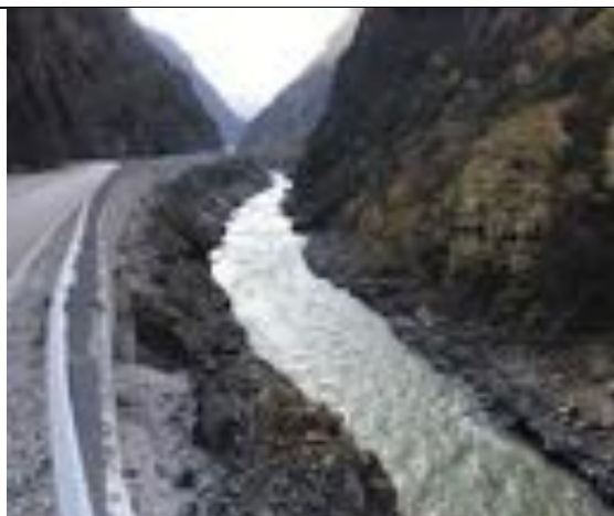
Photo 153. I-20 Devoll river, typical river morphology in the stretch to be dewatered, downstream of Moglice
