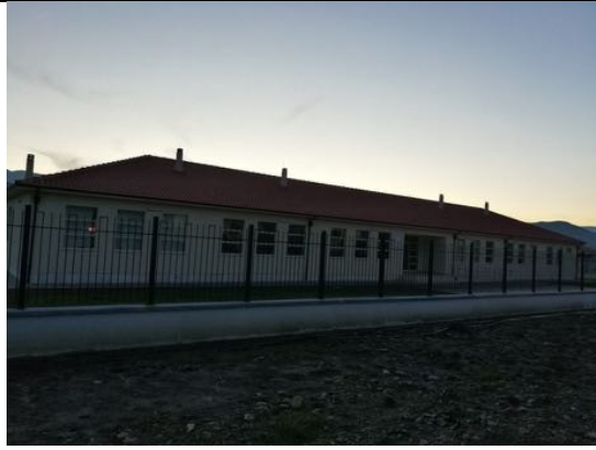
Photo 39. I-9 Replacement Drize School
