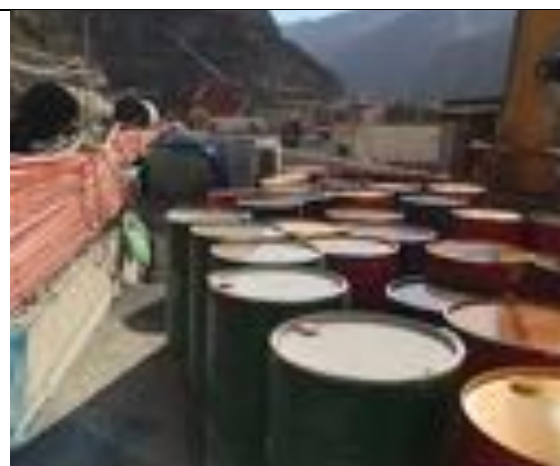
Photo 135. I-18 Oil drums at Moglice tunneling site with untidy site in background
