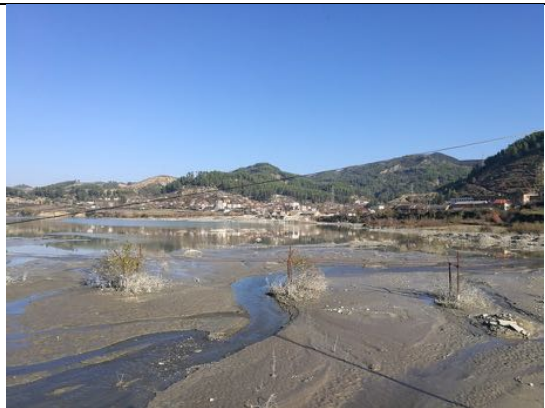
Photo 66. I-10 The old Trashovice Bridge (now Abandoned)
