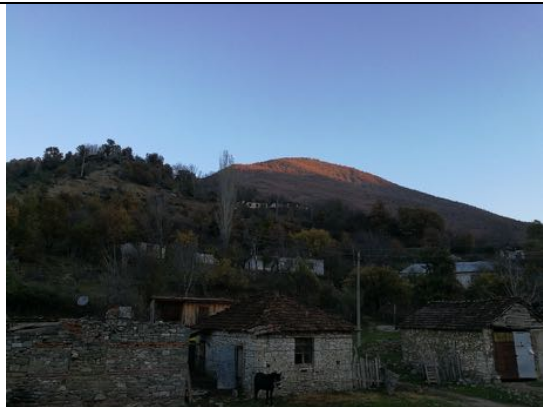
Photo 52. I-10 Houses to be Inundated in Nikollare Village
