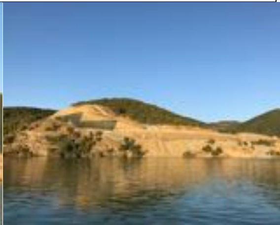
Photo 110. I-16 Erosion prevention measures on Banje north shore road, as seen from reservoir (2)
