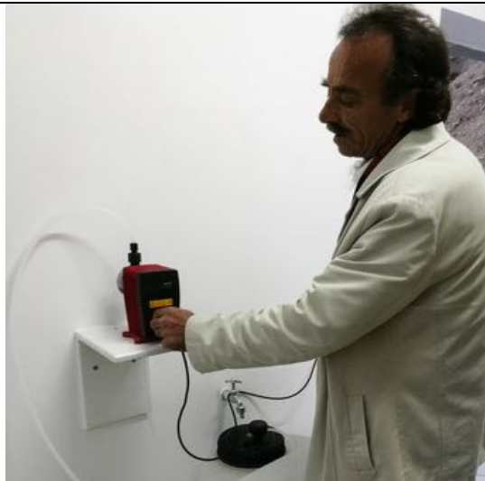
Photo 25. I-7 New Water Supply for Cejure and Drize
