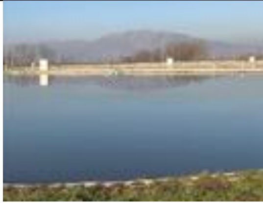
Photo 125. I-17 KfW-financed WWTP on the Korce Plain, far upstream of the project
