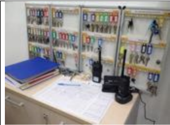
Photo 68. I-12 Access control in Banjë power house
