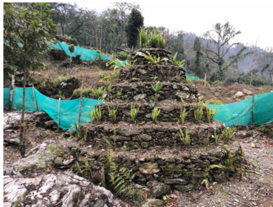
Photo 3: Works in Progress at Butterfly Reserve
