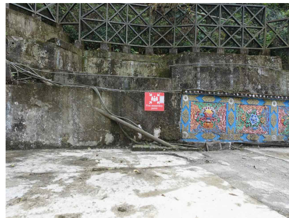
Photo 36: Fire Assembly Point Signage
