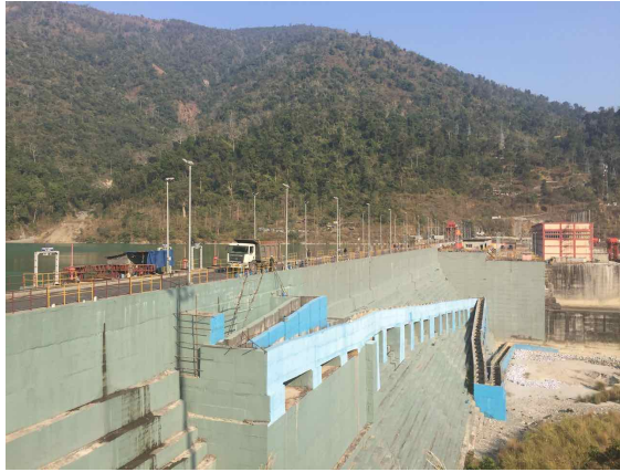
Photo 97: Fish Passage on Teesta Low Dam IV
