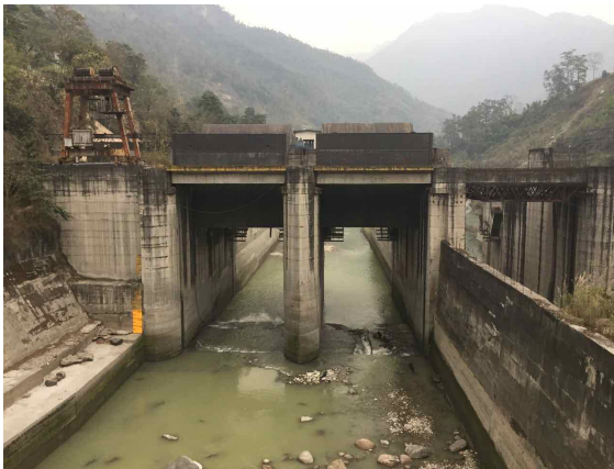
Photo 89: Downstream Teesta-VI Dam with Algae Growth Indicating Water Level Fluctuations during Dry Season
