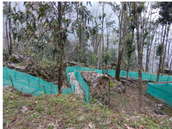
Photo 4: Works in Progress at Butterfly Reserve 2
