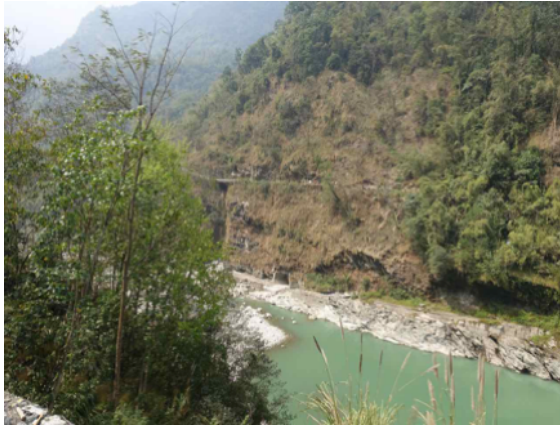
Photo 19: Downstream View from Dam Showing Road on Right Bank to Lum Village
