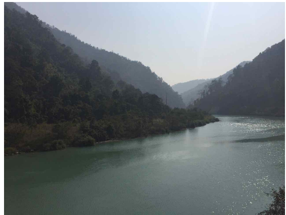
Photo 96: Downstream Reservoir of Teesta Low Dam III
