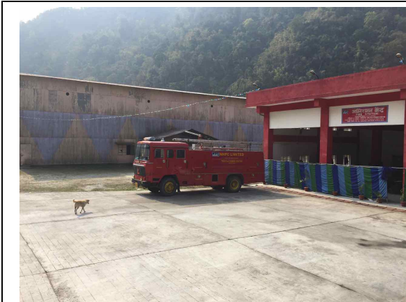
Photo 37: Fire Station at Powerhouse
