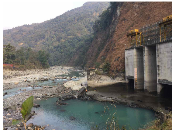
Photo 42: Repairs at Tailrace
