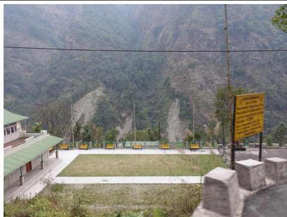
Photo 5: Landslides on Right Bank of Reservoir
