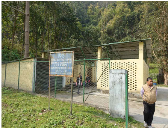
Photo 59: Solid Waste Separation & Composting Plant
