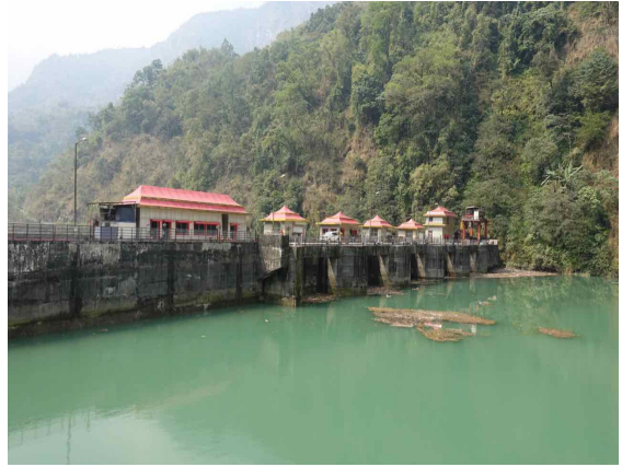
Photo 8: Debris in Reservoir at Dam
