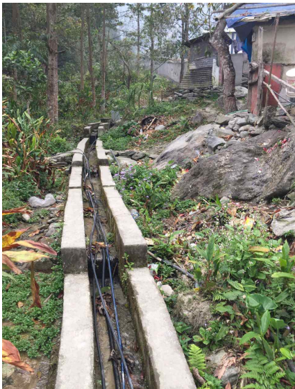
Photo 51: Drainage and Water Supply in Village next to Powerhouse Colony
