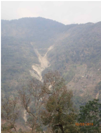
Photo 21: Steep Slopes and Landslide on Right Bank between Dam and Powerhouse
