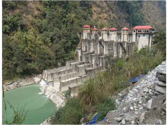
Photo 10: Dam Showing Multiple Water Discharge Points, with Road Stabilization Works in Foreground
