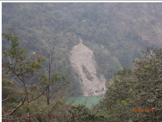
Photo 6: Landslide on Right Bank of Reservoir
