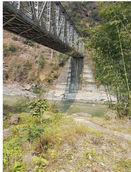
Photo 22: Water Quality Sampling Location near Adit III
