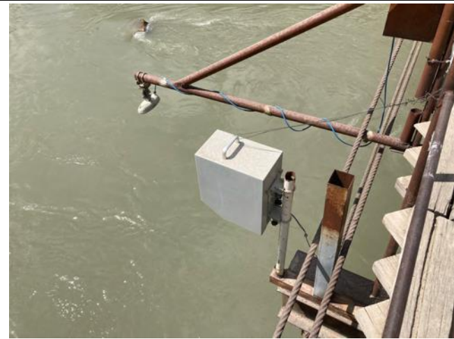
Photo 28: Flow gauge at old bridge
