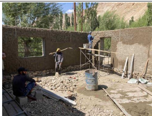
Photo 23: New home for family resettled from flood zone
