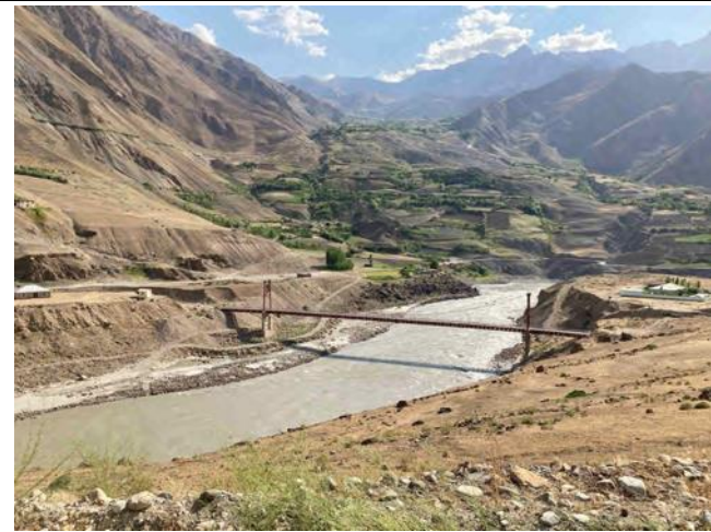
Photo 3: Downstream border crossing into Afghanistan over Panj River
