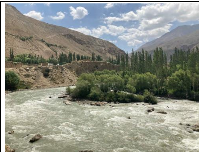
Photo 39: Intake area from downstream
