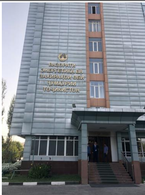
Photo 13: Ministry of Energy and Water Resources, Dushanbe
