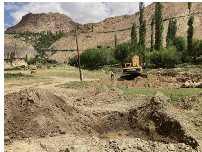
Photo 49: Topsoil excavation at intake
