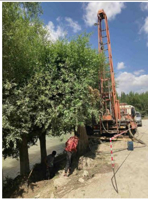
Photo 32: Test drilling at bridge upstream of intake
