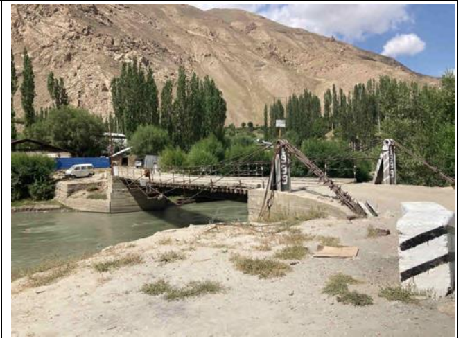
Photo 27: Old bridge upstream of intake
