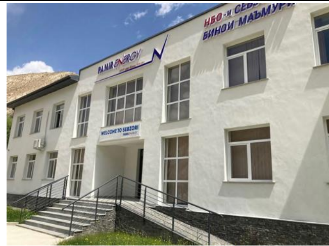
Photo 46: PEC Sebzor administrative building
