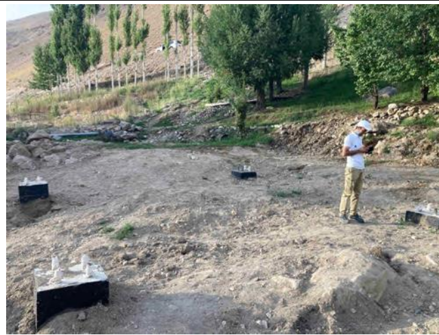
Photo 74: Transmission line tower foundations in Upper Chagev
