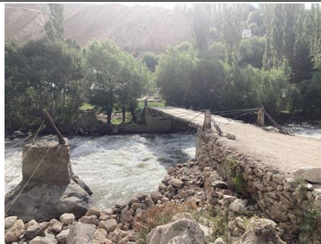
Photo 53: Bridge to Sebzor village on left bank near powerhouse
