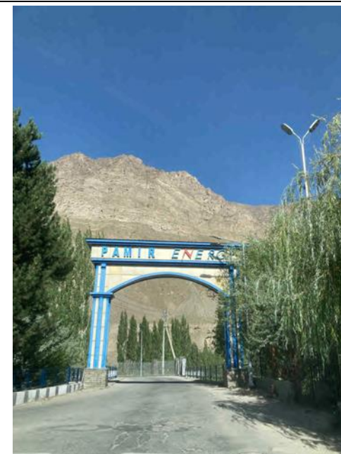
Photo 15: Gate to PEC main office and Khorog HPP
