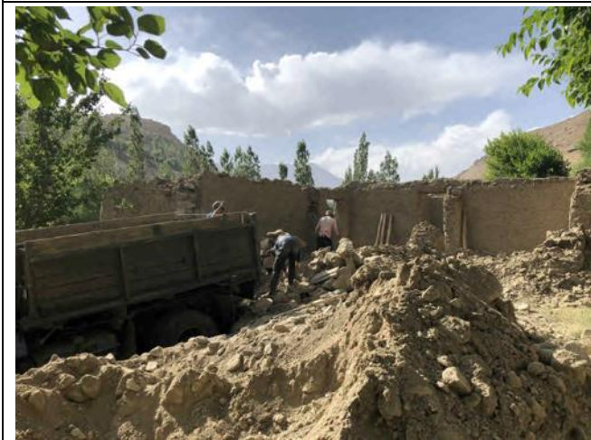
Photo 58: Demolishing of resettled family home at powerhouse
