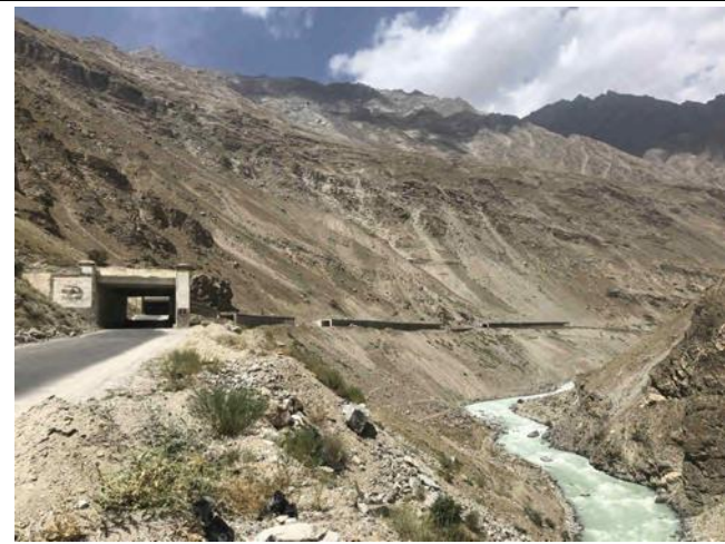
Photo 7: Galleries to protect Pamir Highway in Gunt valley from rockfall
