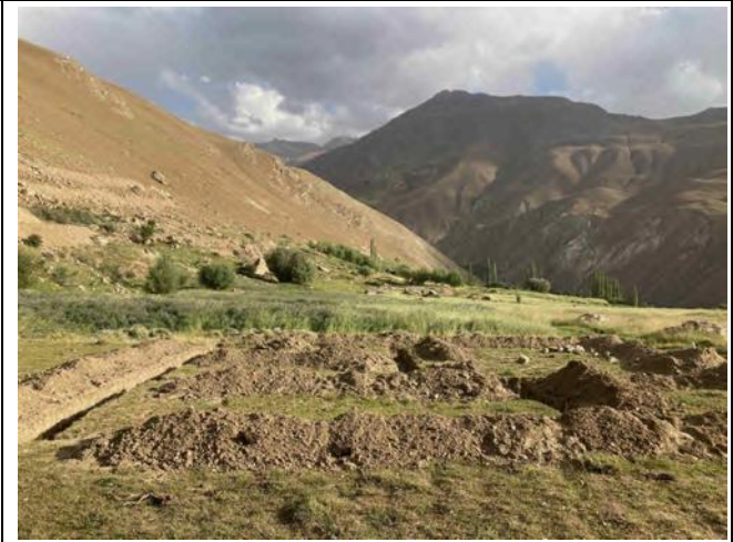
Photo 69: New home site preparation in Upper Chagev
