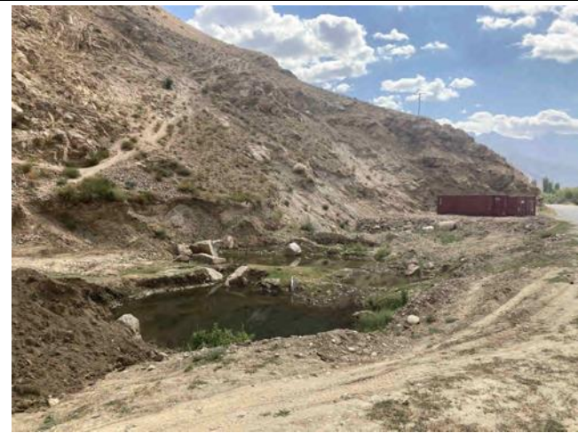
Photo 25: Spoil disposal area 1
