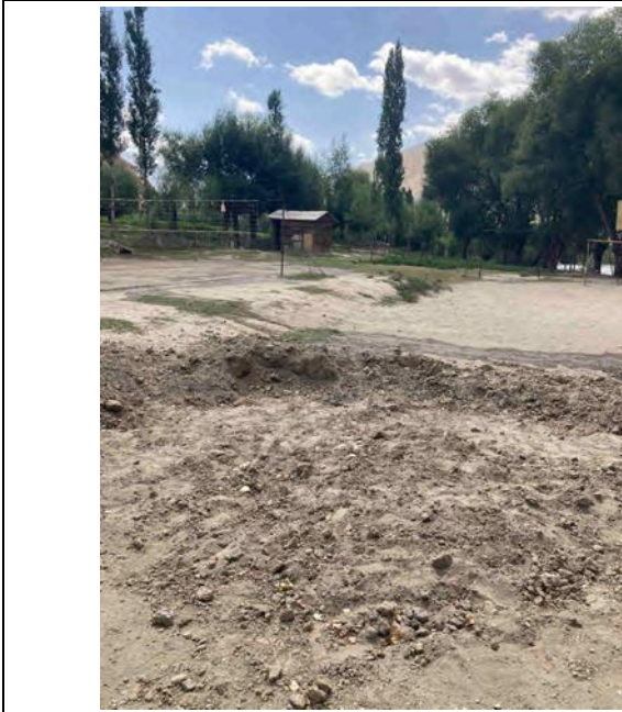
Photo 31: Refilled test pit at school
