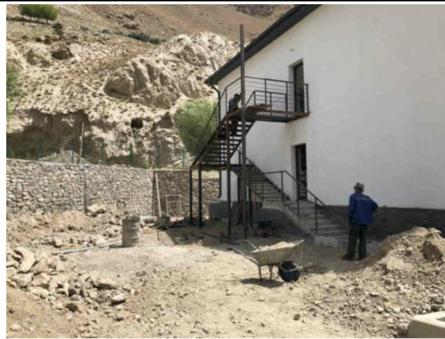
Photo 47: Finishing works at PEC Sebzor building
