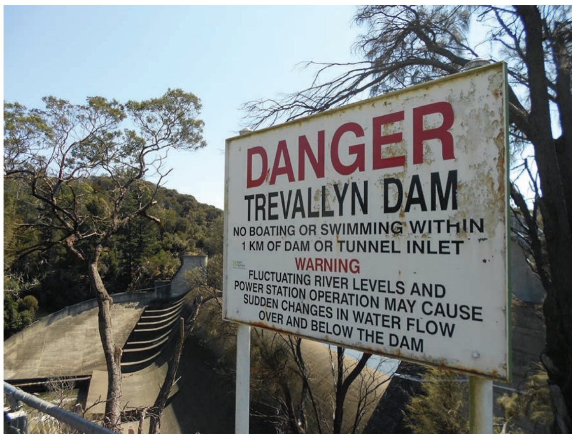
Figure 8. Public safety around dams: Trevallyn, Australia Photo Credit: Joerg Hartmann
