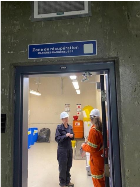
Photo 7: Waste separation room
