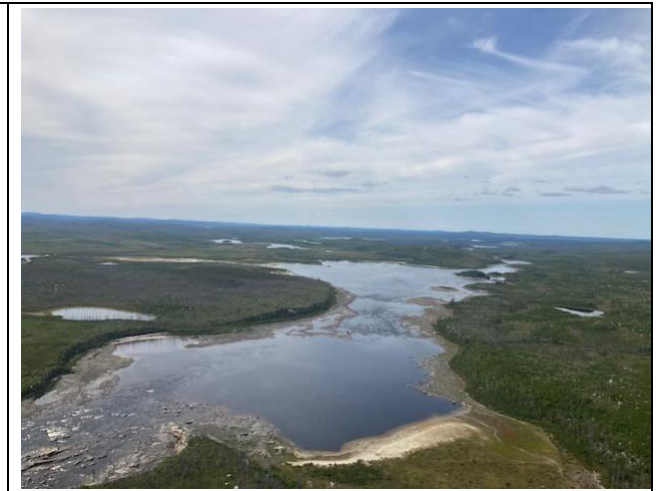
Photo 105: Reduced flow section of the Rupert River
