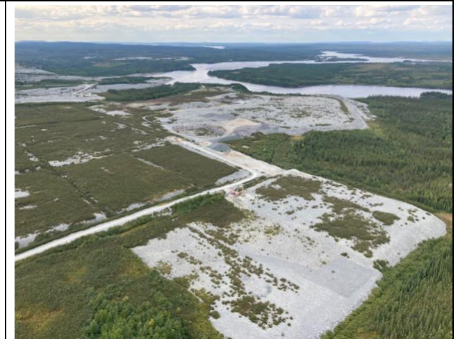
Photo 6: Partially revegetated work areas next to Eastmain-1a, view towards Eastmain River
