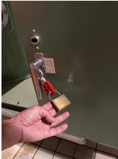
Photo 8: Equipment with personal safety lock
