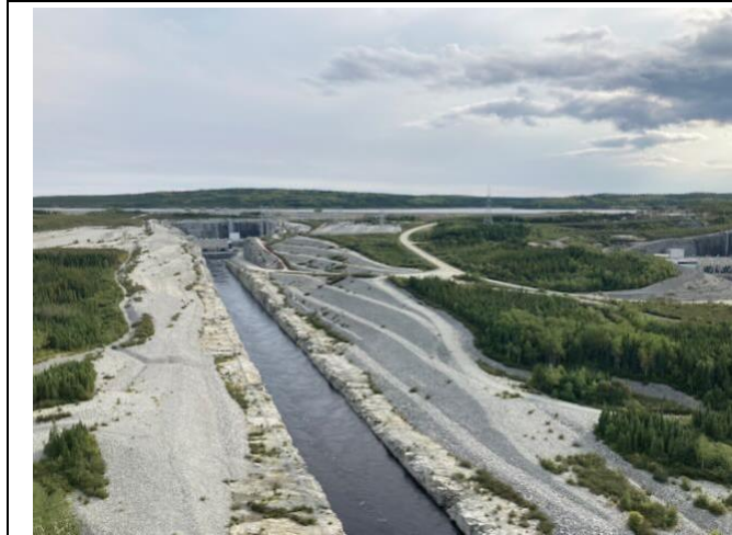
Photo 4: Tailrace of Eastmain-1a
