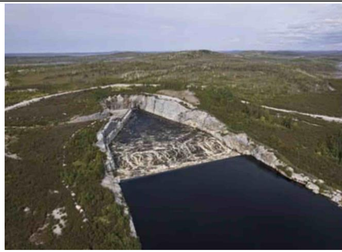
Photo 74: Tommy Neeposh Tunnel intake
