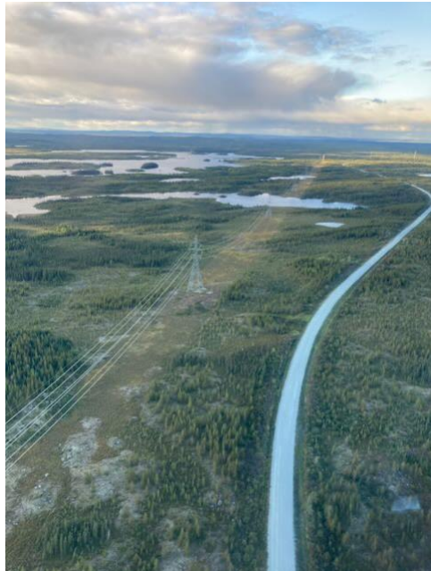
Photo 62: Transmission corridor and road to Eastmain
