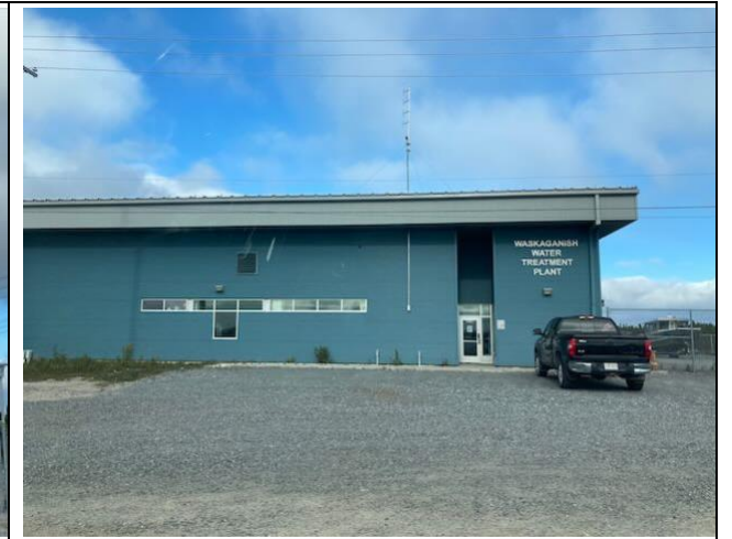
Photo 129: Water treatment plant funded by project
