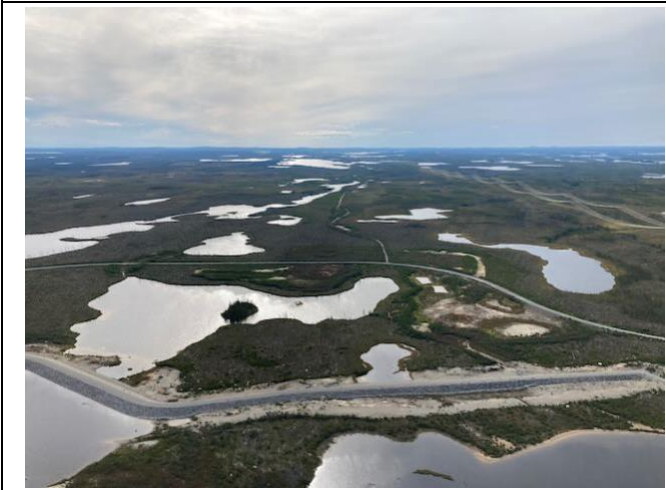
Photo 76: Embankment dikes on Rupert tailbay
