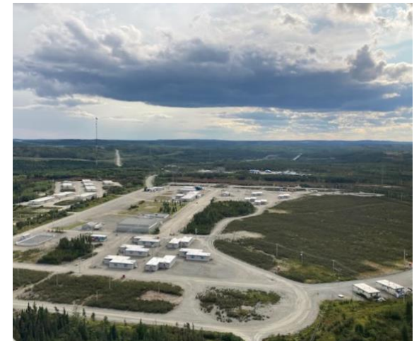
Photo 18: Camp with rehabilitated part on right
