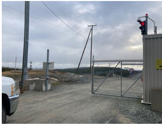
Photo 41: Entrance controls at Eastmain dam
