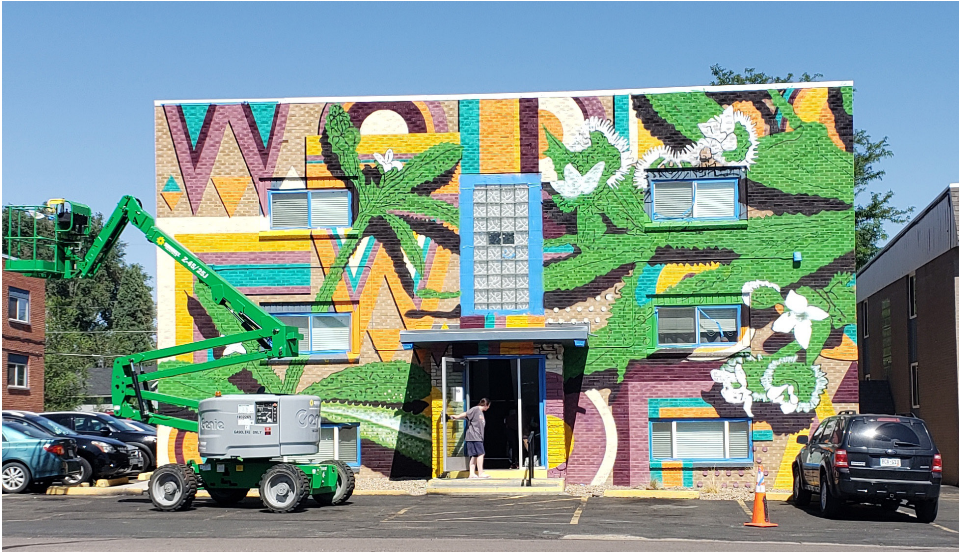
“Cleavers” 24' x 48' Lamar Station Apartments Building F
