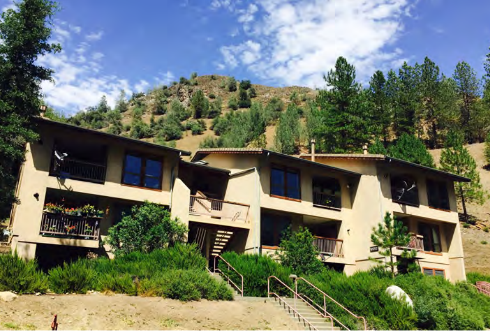
Homes in the Rancheria Flat area of El Portal.
