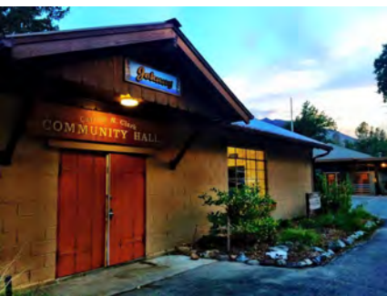
The community hall in El Portal, on Foresta Road between the post office and gas station.
