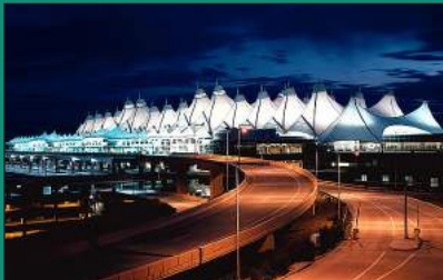
22 Denver International Airport
