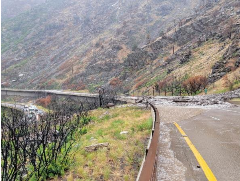
(Fig. 2: Debris Flow Covering Westbound Lane of I-70) 2
