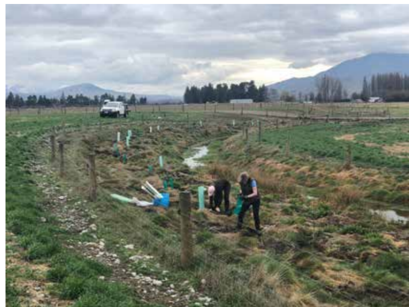
Figure 5-4. Planting trees in a fenced-off riparian zone, Omarama Station.
