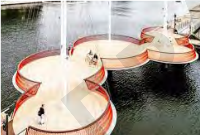
Circle Bridge, Denmark
