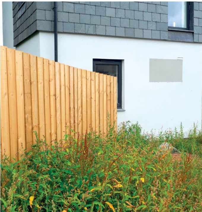
Image 5: Church Road is currently in construction, and although some green infrastructure features are yet to be established, it is clear from the BwN site photos that Coastline Housing commitment to manage surface water runoff in part through drainage to soft green verges is evident in the built out scheme
