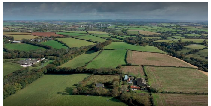
Image 3: Aerial View of the Langarth Garden Village site with the proposed Governs Park in the foreground. The Park will fulfil the function of a Suitable Alternative Natural Green Space and will be managed for biodiversity and recreational objectives
