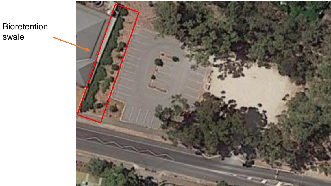
Figure 3: The study area and its surrounds with Stage 1 (consisting of half the planned carpark and the bioretention swale) completed, prior to implementation of the other planned features.
