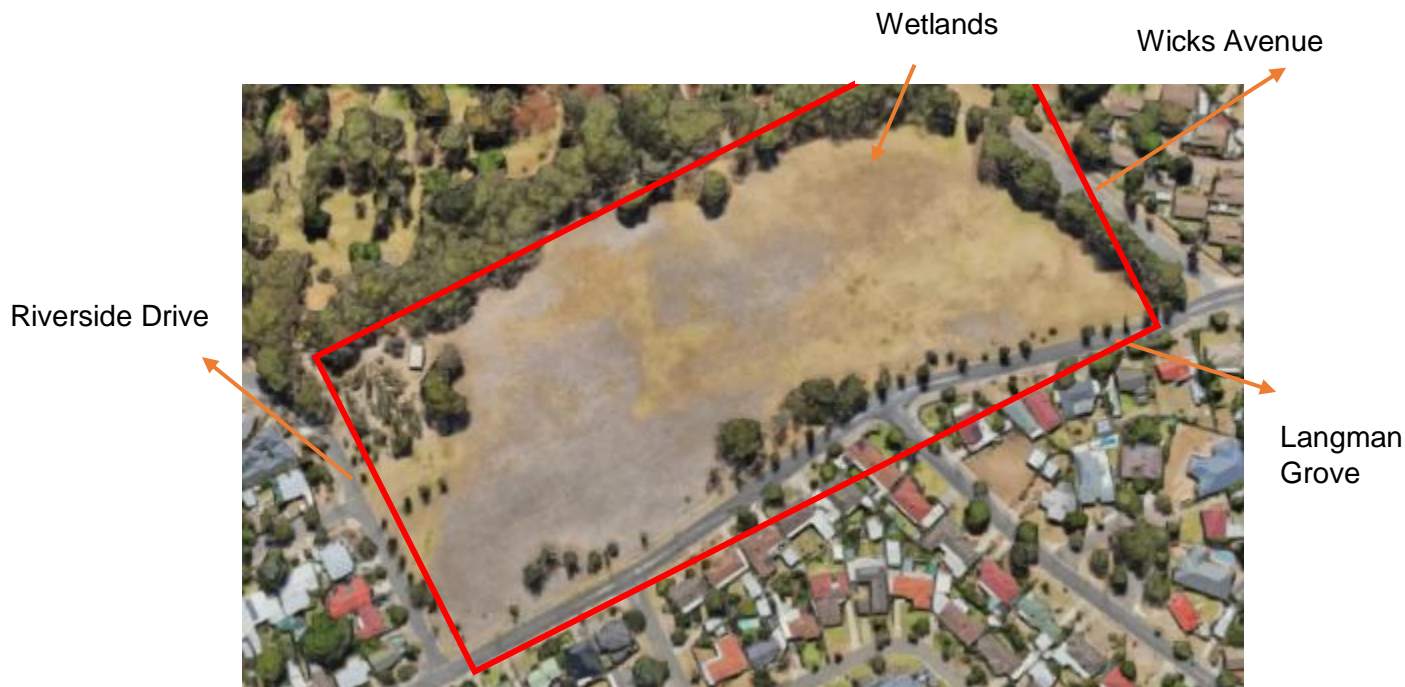
Figure 4: The study area and its surrounds prior to implementation of all WSUD and GI features.
