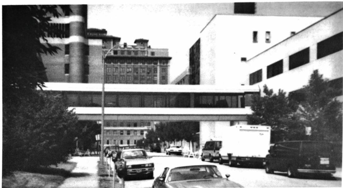
The Dental School is almost hidden by the new overpass constructed by the School of Medicine between the Medical Dorm and the Radiology Building (Old A and P bakery). Cost of overpass has been estimated at almost a million dollars. (This picture taken from parking lot east of the dorm.)
