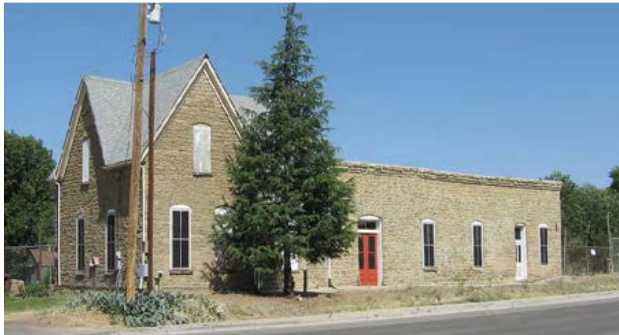
The Silver City Waterworks Building.
