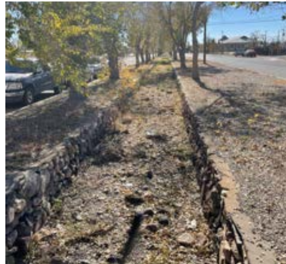
The arroyo provides a great focal point and a connection from Town Hall towards the Chino Club.
