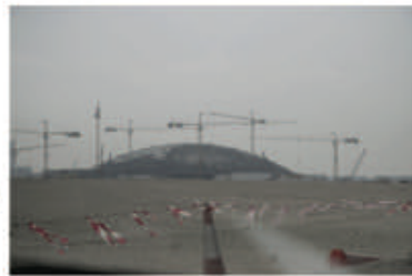
Louvre Museum Construction, Abu Dhabi, March 2015.
