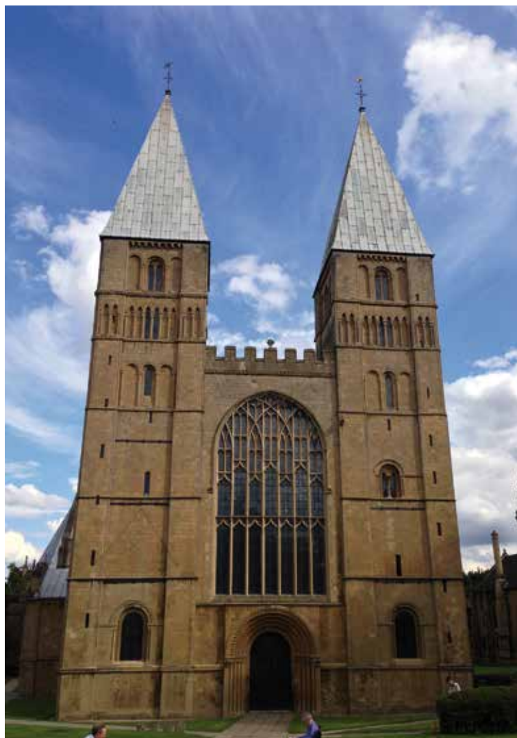
West front of Southwell Minster; severe Romanesque of the towers and west door contrasts with later Perpendicular west window and battlement
