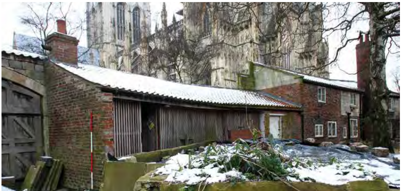
Below: Outbuildings and generator cellar, looking SE
