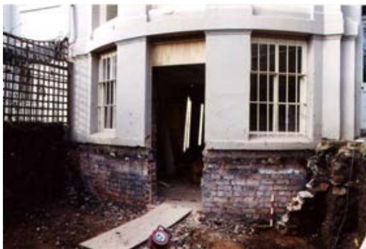
Watching Brief – view of the house after removal of brick vault
