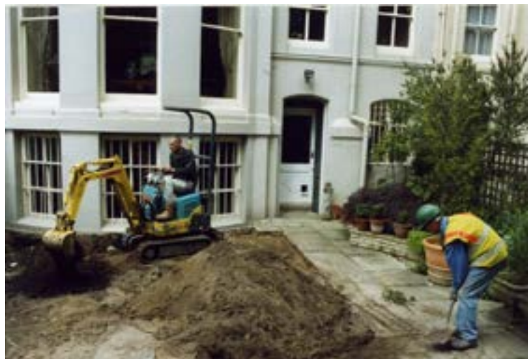
Removing garden soil by machine
