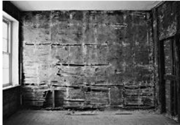
Post-medieval lath and plaster on an internal wall
