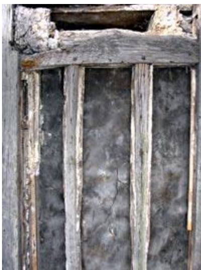
15th century window mullions
