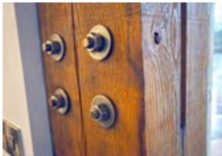
A portal-style oak frame has been used to provide an uncluttered interior to take advantage of the lakeside views. The combination of oak, steel and glass, gives the low-lying structure a distinctly contemporary look.
