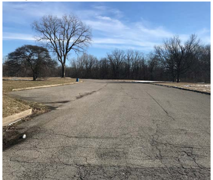
existing loop road
