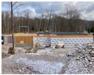
Ready For Floor Trusses
