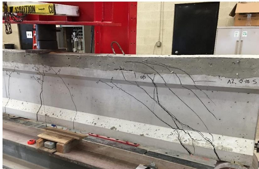
Figure 8: Girder A2s failure
