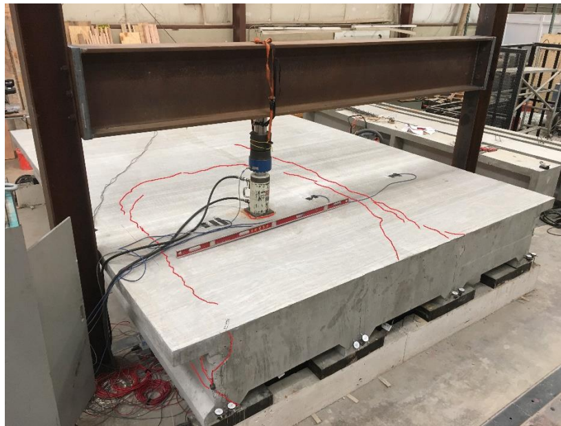
Figure 13: Cracking in scale bridge deck after testing
