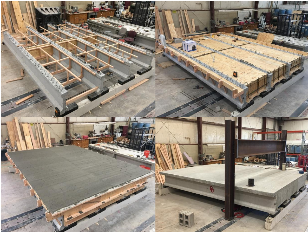
Figure 6: Scale bridge construction progress
