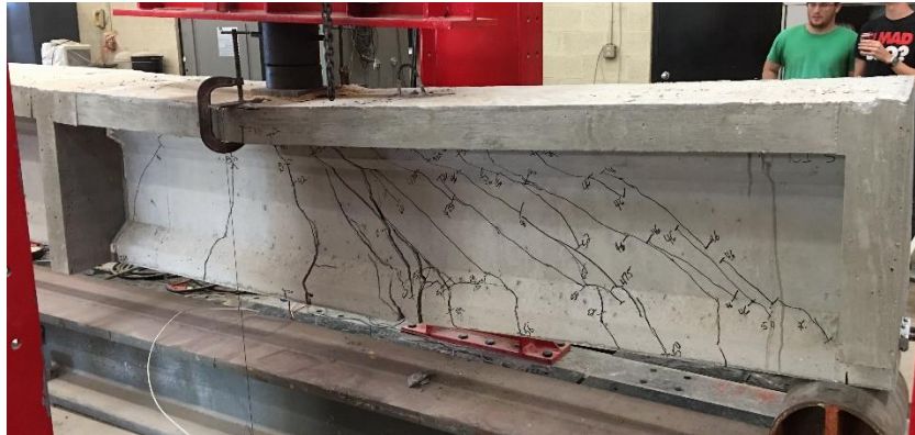
Figure 9: Girder C1s failure
