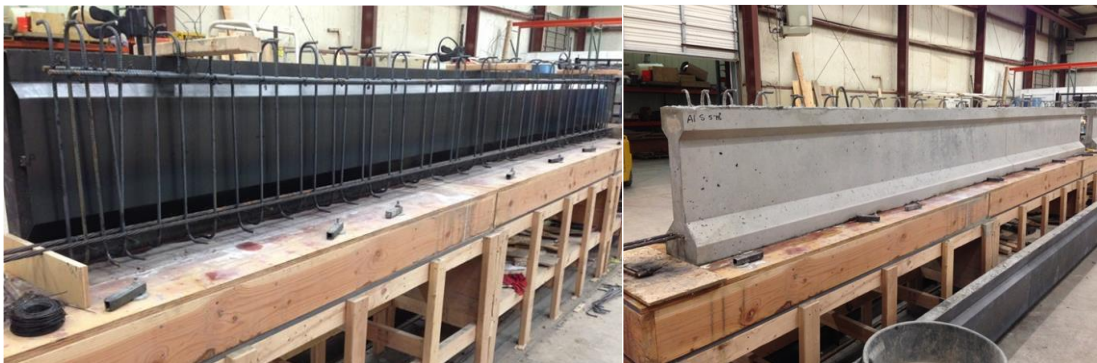
Figure 4: Scale girder shear steel and prestressing strands (left) and completed girder prior to de-tensioning (right)
