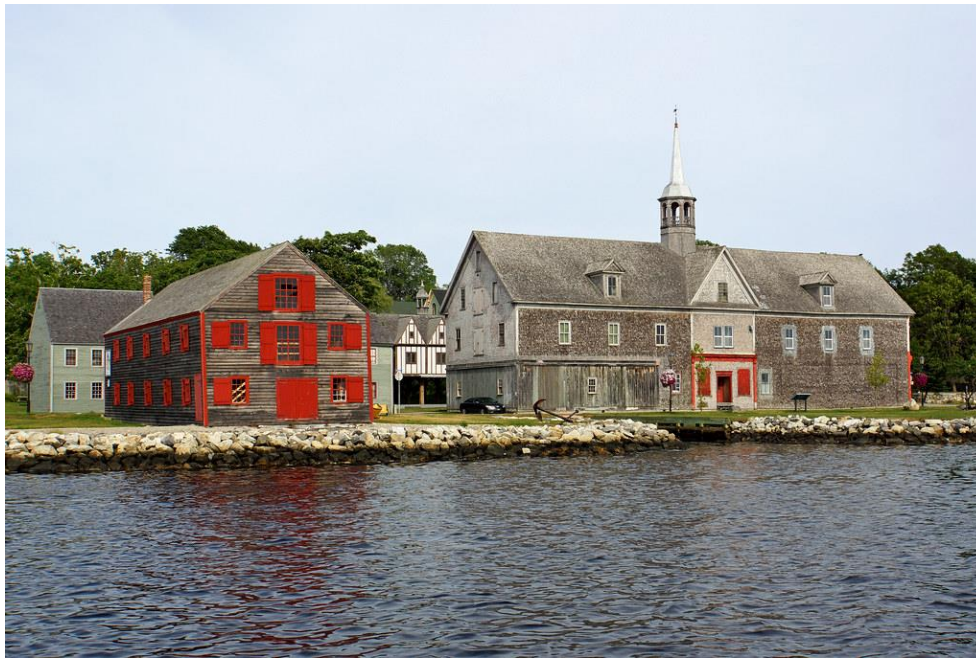
Figure 3. Shelburne’s historic waterfront. Note armour stone along the shoreline. (Dennis Jarvis. Creative Commons. CC BY-SA 2.0)
