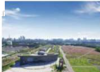
Because the Proteus technology can be installed underground, a plant in Seoul, South Korea was able to put a park above the treatment facility.
