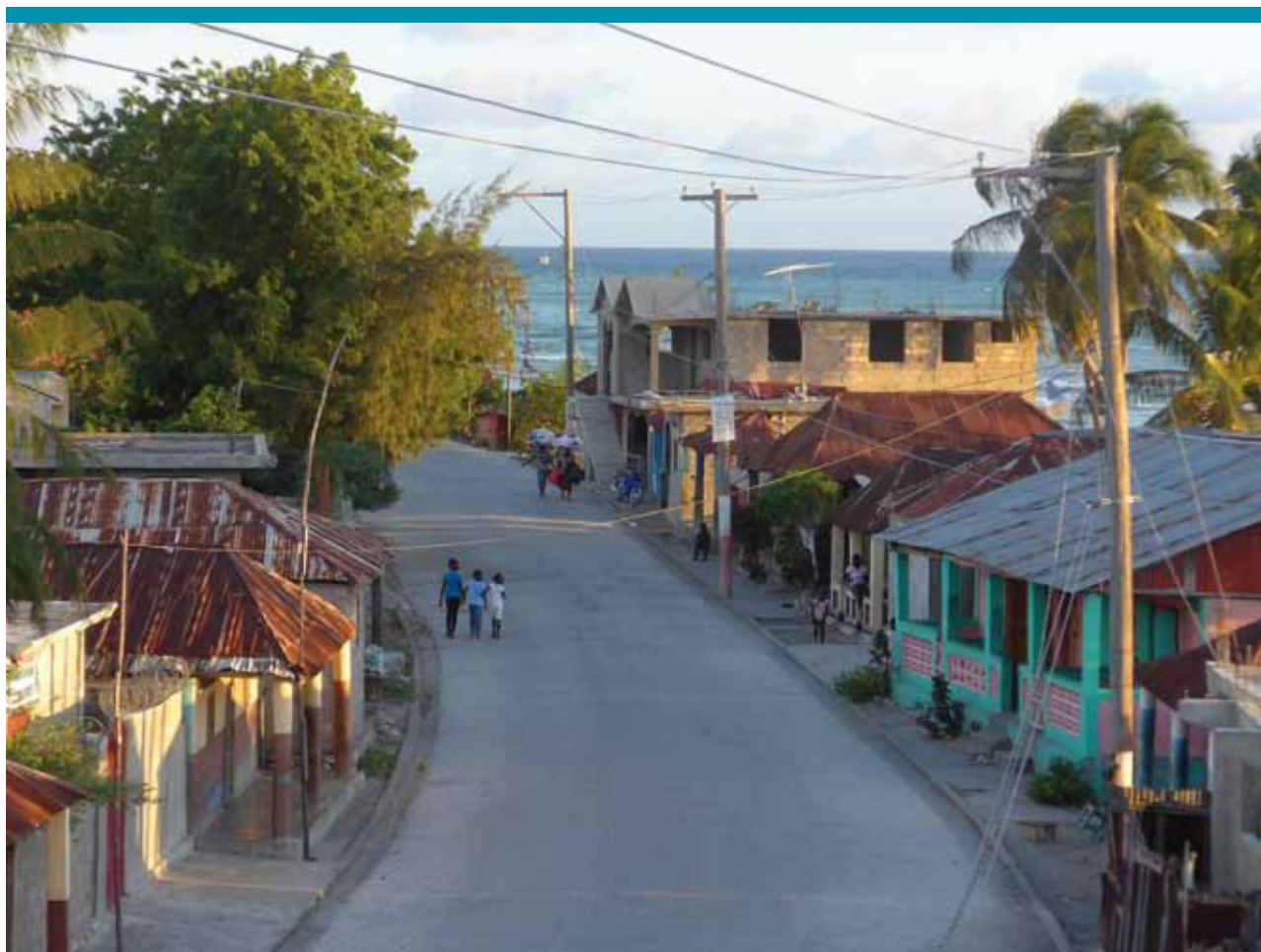
In Haiti, 19 US-based electric co-operatives and 37 volunteer linemen worked with the National Rural Electric Co-operative Association (NRECA) International to help build Haiti's first electric co-operative. The possibilities are now endless for three towns in the southwestern region of the country, because a better life starts with power.
