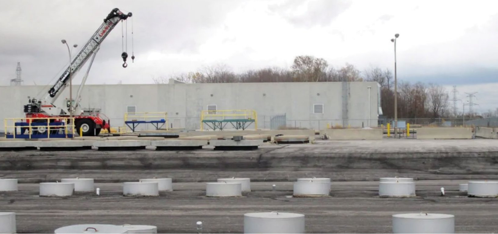
Figure 50. Rows of chambers holding intermediate level radioactive waste, seen here in 2013 at the Bruce Power nuclear complex near Kincardine, Ontario (Source: CBC)
