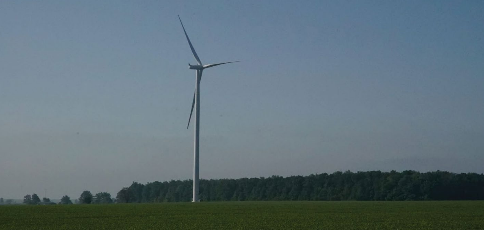
Figure 27: SNGRDC Wind Turbine (photo credit: Power to the People, Real World Media)
