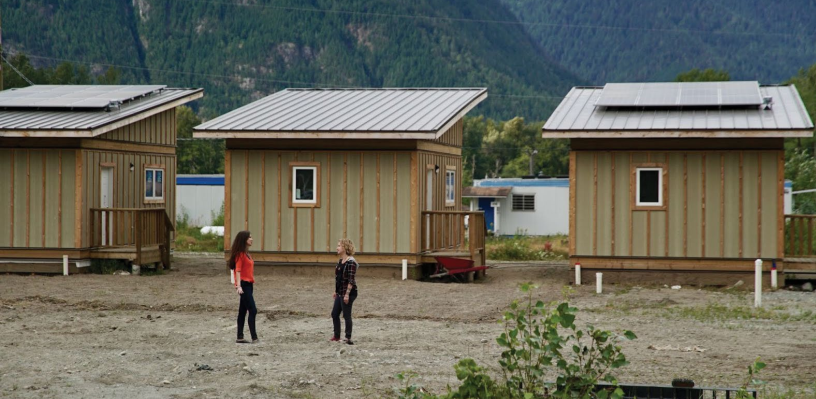
Figure 62: Sustainable Housing in Bella Coola (photo credit: Power to the People, Real World Media)
