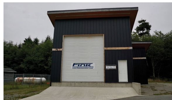
Figure 42: Haida Gwaii Biomass Facility (photo credit: Power to the People, Real World Media)
