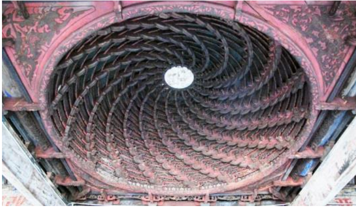
Fig. 4. Spiral zaojing (chicken-cage type) in the opera stage of Yu'shi Ancestral Temple, in Ninghai, rebuilt in 1911. Height: 1.46m; Diameter: 3.8m. Ref. ZJ-03 © Jingxian Ye
