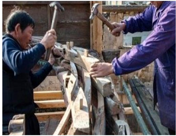
Fig. 25. Hammering of the reassembled zaojing © Xiaodong Chai
