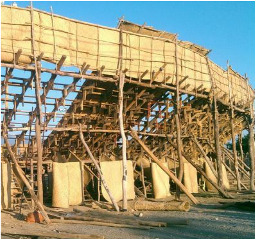
Fig. 2. Building process ( www.ecosdelacosta.mx )
