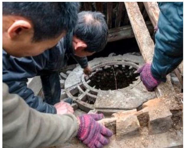
Fig. 17. Removal of top plates © Xiaodong Chai
