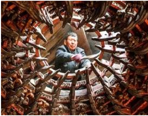
Fig. 18. Hammering of the zaojing © Xiaodong Chai
