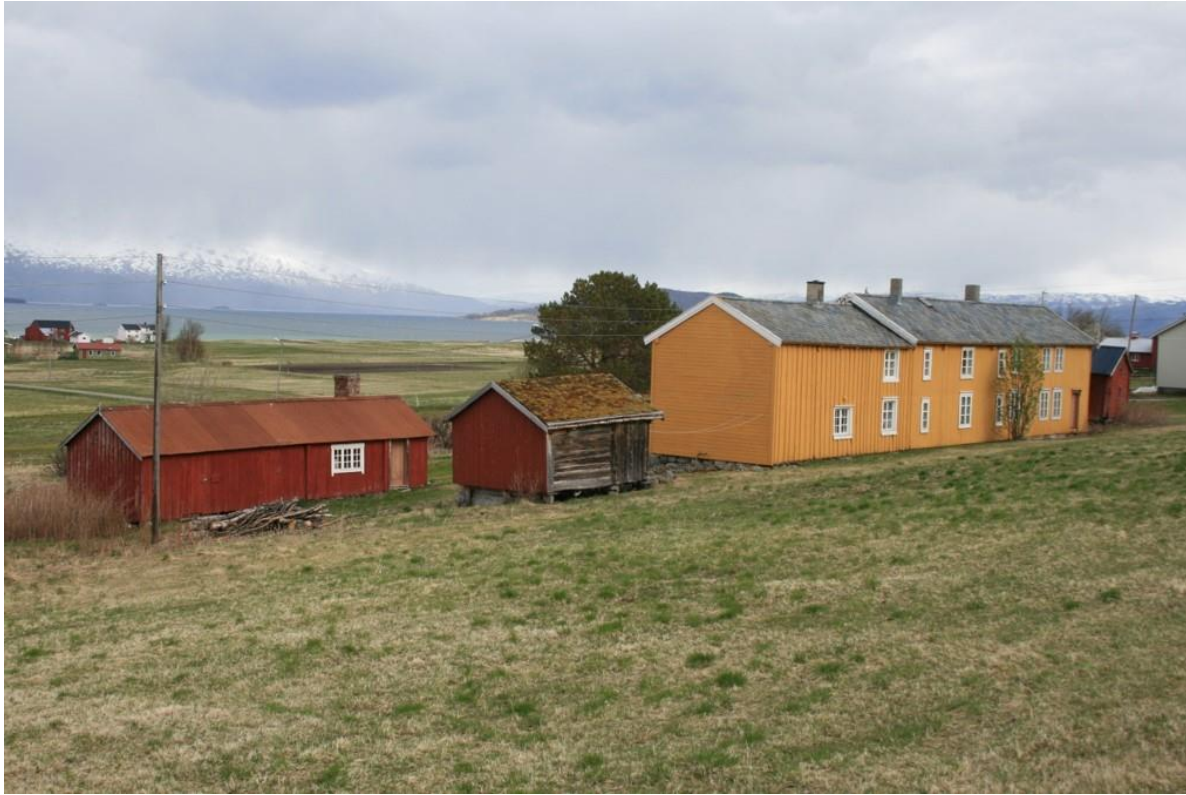
Fig. 1. The Ljones farm in Salten. All main buildings are orientated towards the predominant wind. From left the old living house built 1606, later used as smokehouse, a storhouse built 1589, the living house from mid 18th century and onwards. The living house has a timber frame «sval» in both ends of the building, which functions as an outhouse and climate zones, protecting the log construction. The «sval» can only be reached trough the door in the longwall, and there are no internal connection to the living rooms made in log construction. All Photographs by Author.
