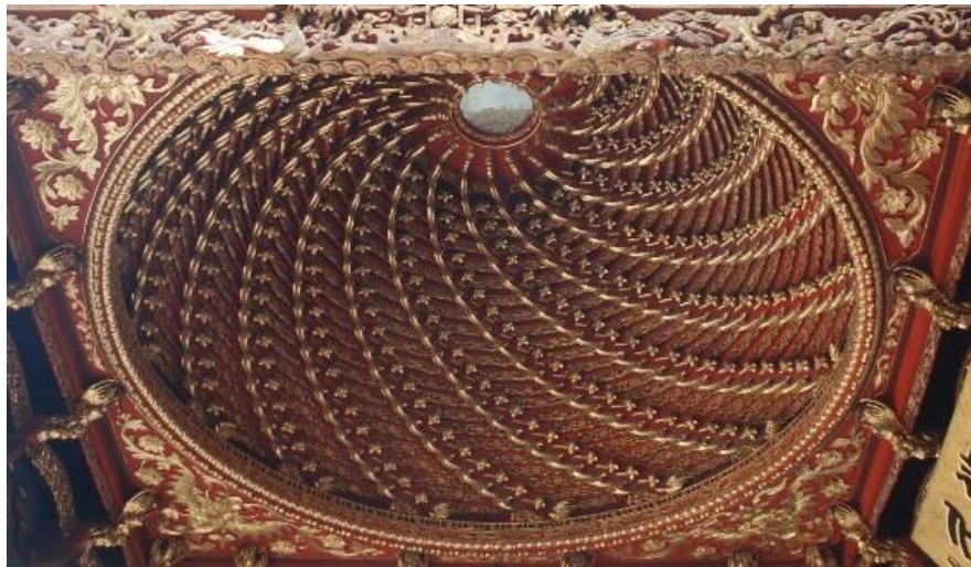
Fig. 3. Spiral zaojing (chicken-cage type) in the opera stage of Qin'shi Ancestral Temple, in Ningbo, built in 1925. Height: approx. 2.25m; Diameter: approx.5m. Ref. ZJ-02 © Jingxian Ye
