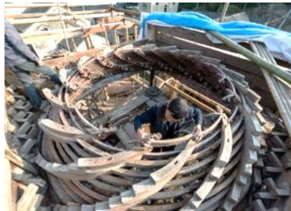
Fig. 26. Close to completion © Xiaodong Chai
