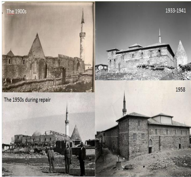
Fig. 5. Repair of façades (VGM Archive)
