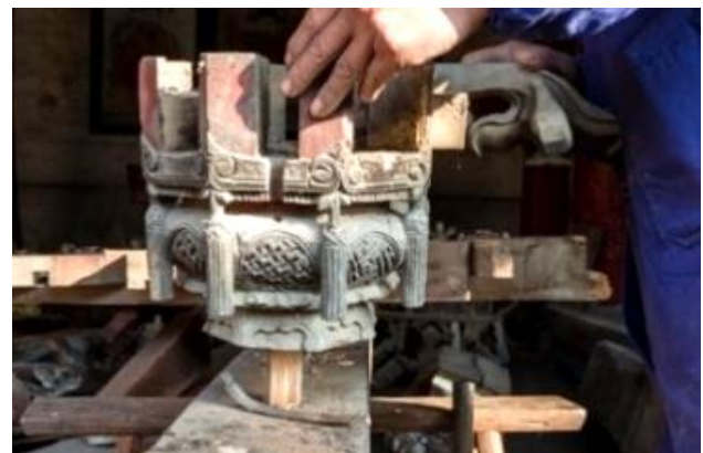
Fig. 23. Manufacturing of new tenon tongue © Xiaodong Chai
