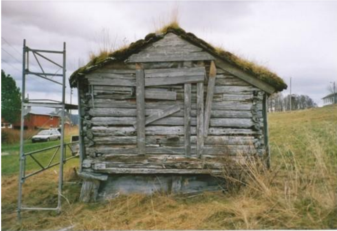
Fig. 4. The Ljoenes storhouse when conservation started, in 2006. Hard wind and rainfall from west had damaged the short wall.
