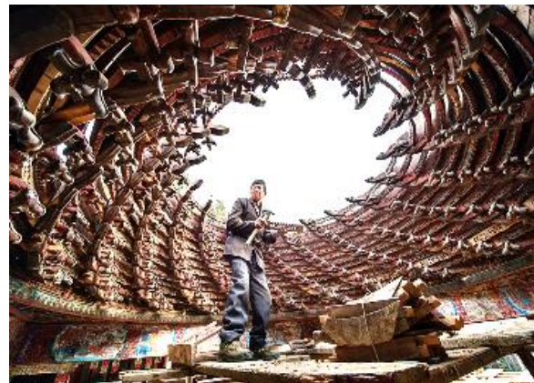
Fig. 27. Close to completion © Xiaodong Chai
