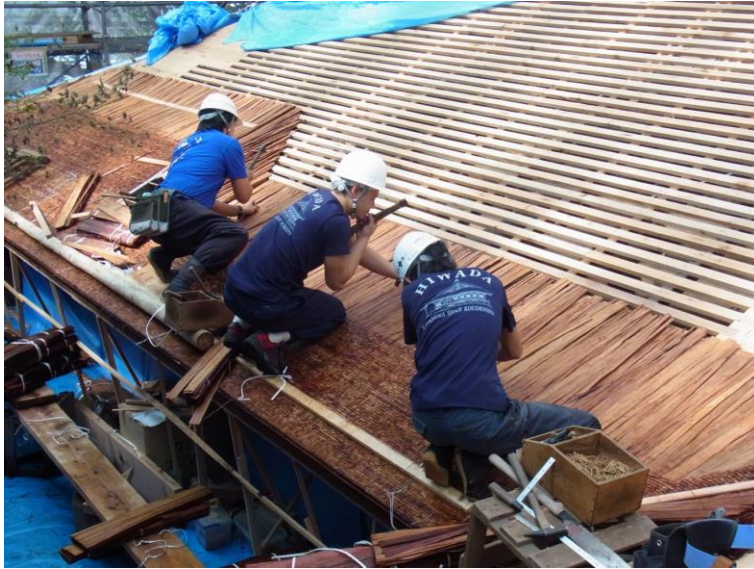
Fig. 1. Roofing with cypress bark shingles (hiwada)
