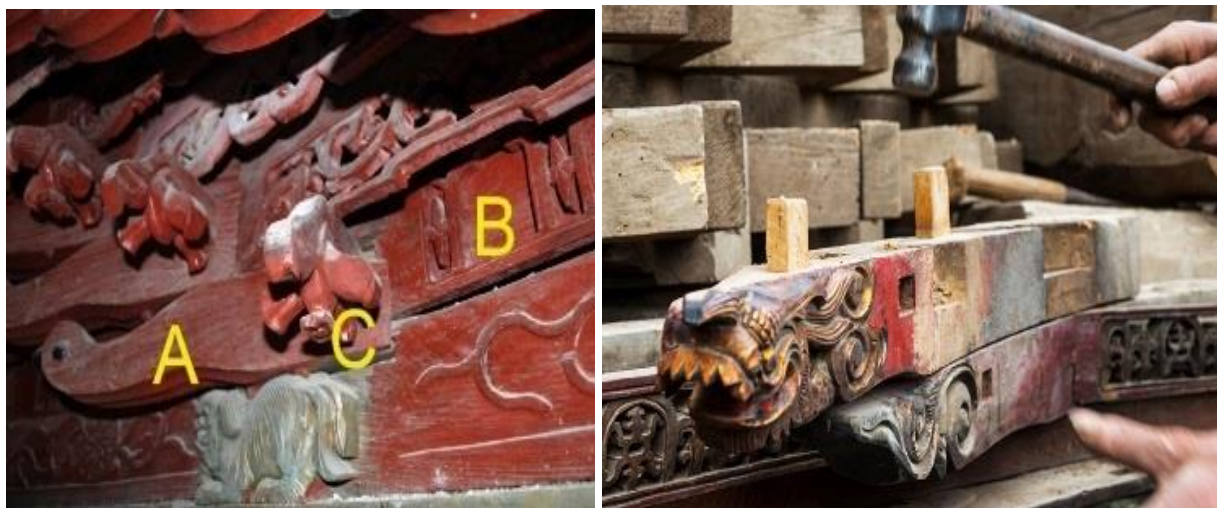
Fig. 13. Components A, B, and C. Spiral zaojing in opera stage of Wei’shi Ancestral Temple, Xiapu Village, Ninghai, built in 1890. Ref. ZJ-04. © Jingxian Ye
