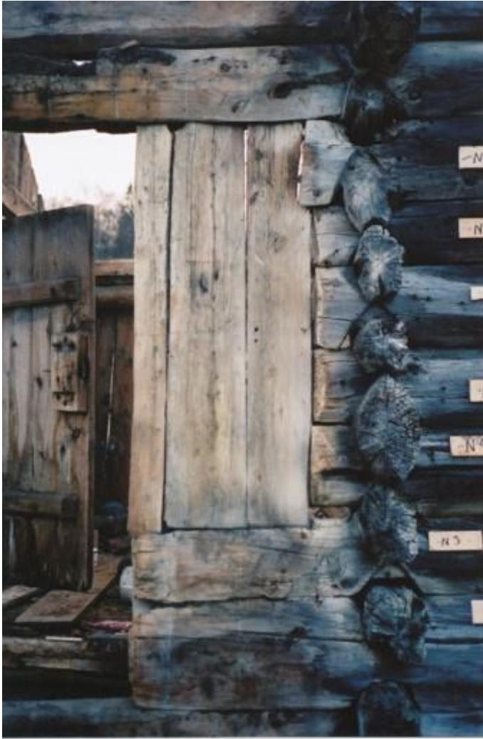
Fig. 5. Details of the Ljones storhouse: The longwall with the log construction to the right and the lighter and more airy entrance and storage room to the left.
