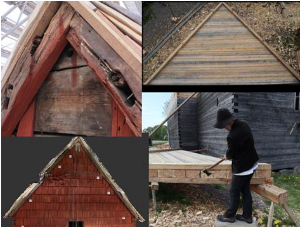
Fig. 6. To the left, above a detail of the gable and the rafters with oblong holes. Left below screendump of 3D model by Camilla Melin of the barns gable. Above right, Ingatorps gable reconstructed on the Södra Råda reconstructions chancel. Photos Karl-Magnus Melin.
