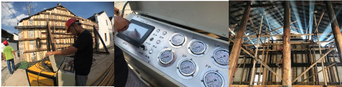
Fig. 8. Wall rectification (self-photography)
