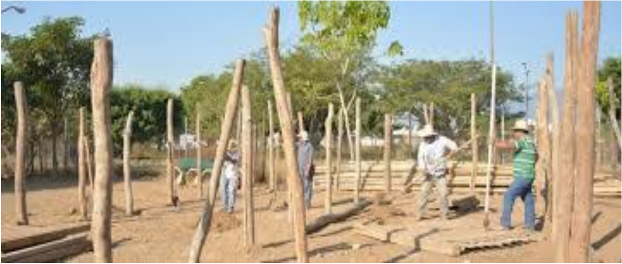
Fig. 5. Dismantling process by the craftman builders ( www.villadealvarez.gob.mx )
