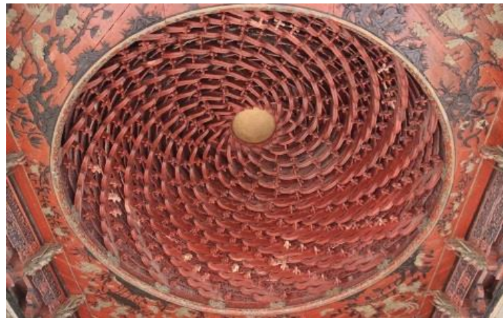
Fig. 5. Spiral zaojing (ox-hair type) in the opera stage of Wei'shi Ancestral Temple, Xiapu Village, in Ninghai, built in 1890. Height: 1.15m; Diameter: 3.3m. Ref. ZJ-04 © Ninghai Lvyou
