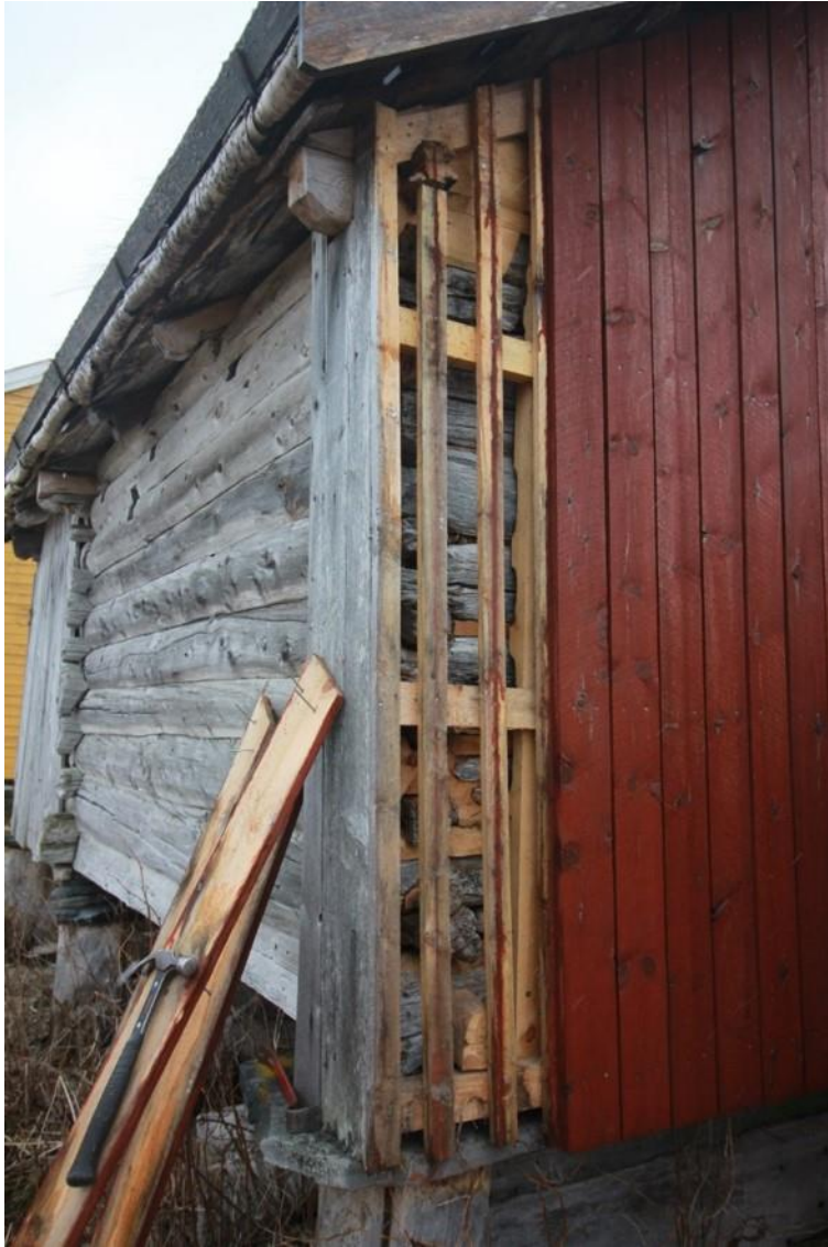
Fig. 6. The storhouse at Ljones was given a climate shell, to protect the damaged short wall against west. In 2017, ten years after the conservation and the boards was put up, the old wall was controlled and it was in a very good condition.
