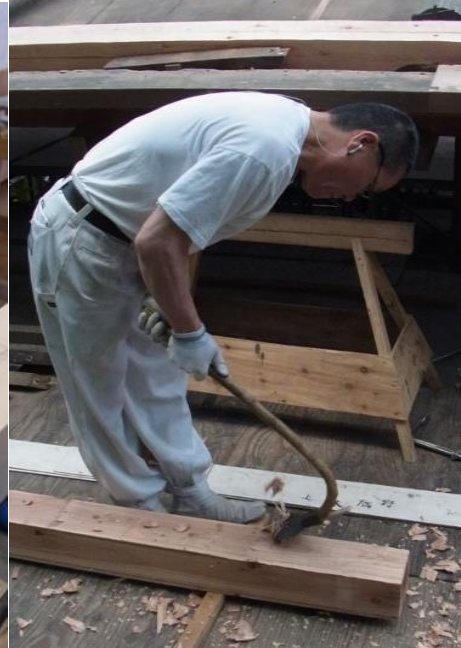
Fig. 4. Finishing with an adze
