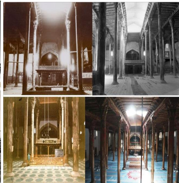
Fig. 6. Repair of inner space (VGM Archive)
