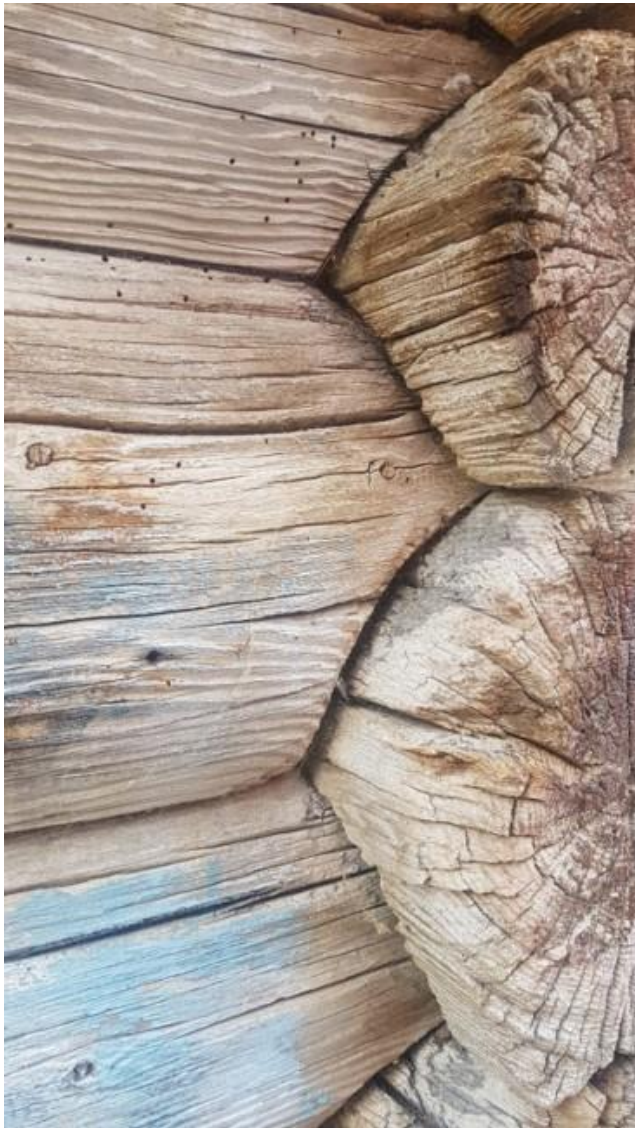
Fig. 7. Typical log hewings from the 16th century in Salten, dated 1564 ac. These log hewings are closely related to the oldest known log hewings in southeast Norway, from before the Black Death.
