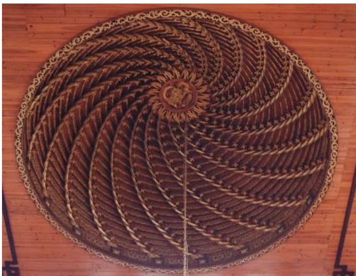
Fig. 6. Spiral zaojing (chicken-cage type) in the main hall of Baoguang Temple, Zhanqi Village, in Yinzhou, built in 2017, by Carpenter Master Liqun Zhang. Height: 2.25m; Diameter: 5.2m. Ref. ZJ-05 © Jingxian Ye
