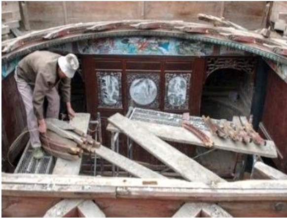
Fig. 20. Same-layer components are tied up © Xiaodong Chai
