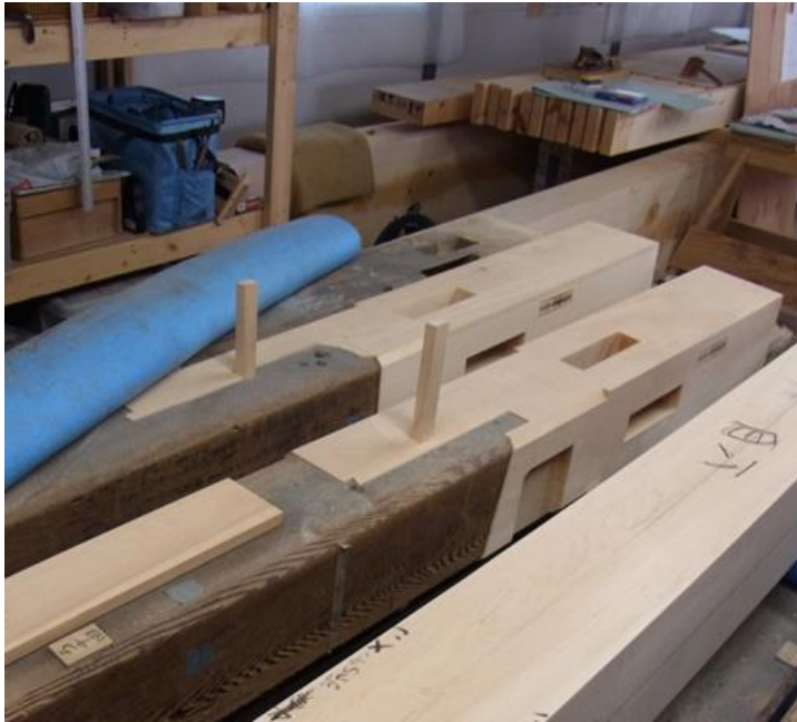
Fig. 3. Repair of pillars with woodwork joints
