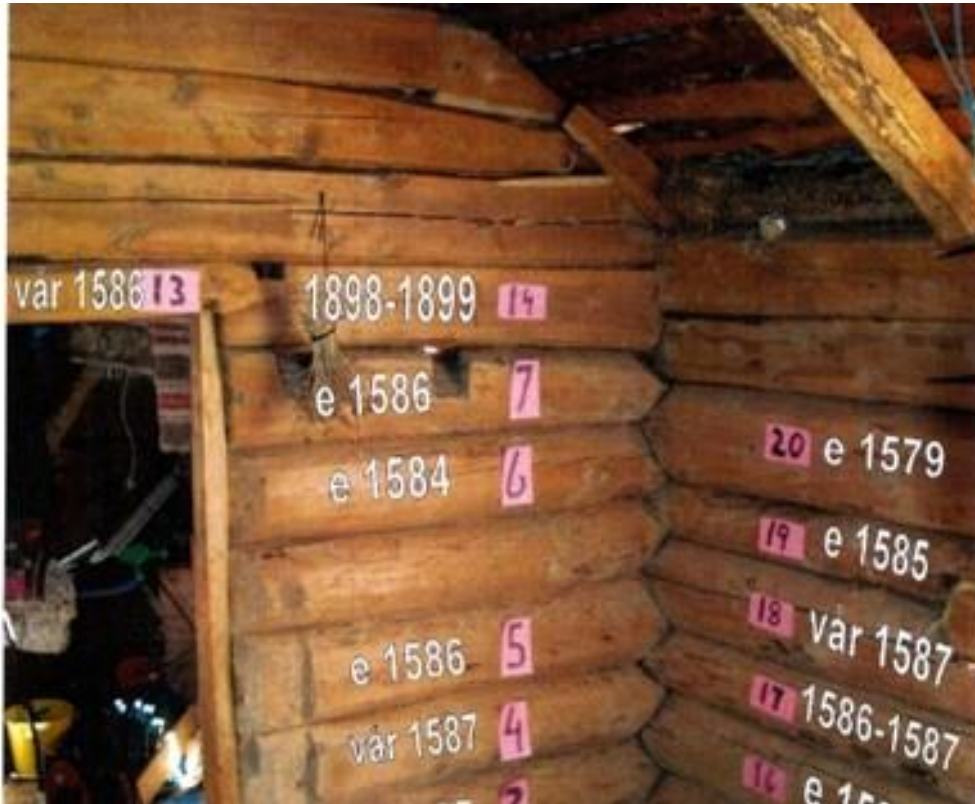
Fig. 3. Examples from the dendrochronological analysis of the Ljones storhouse, built 1589.
